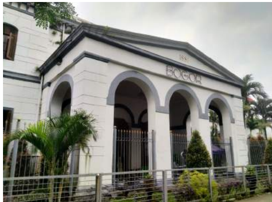
Figure 2.4.4.1: Facade of the heritage building Source: Author (2021)
