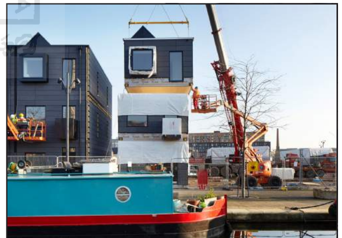
Figure 3.8.3.2: Construction of Modular Home Source: dezeen.com
