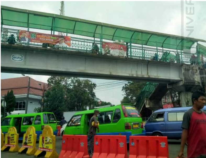
Figure 1.2.4.1: Bridge that connect to the railway station gate Source: Author (2021)
