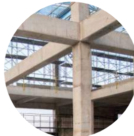
Concrete Column & Beam
