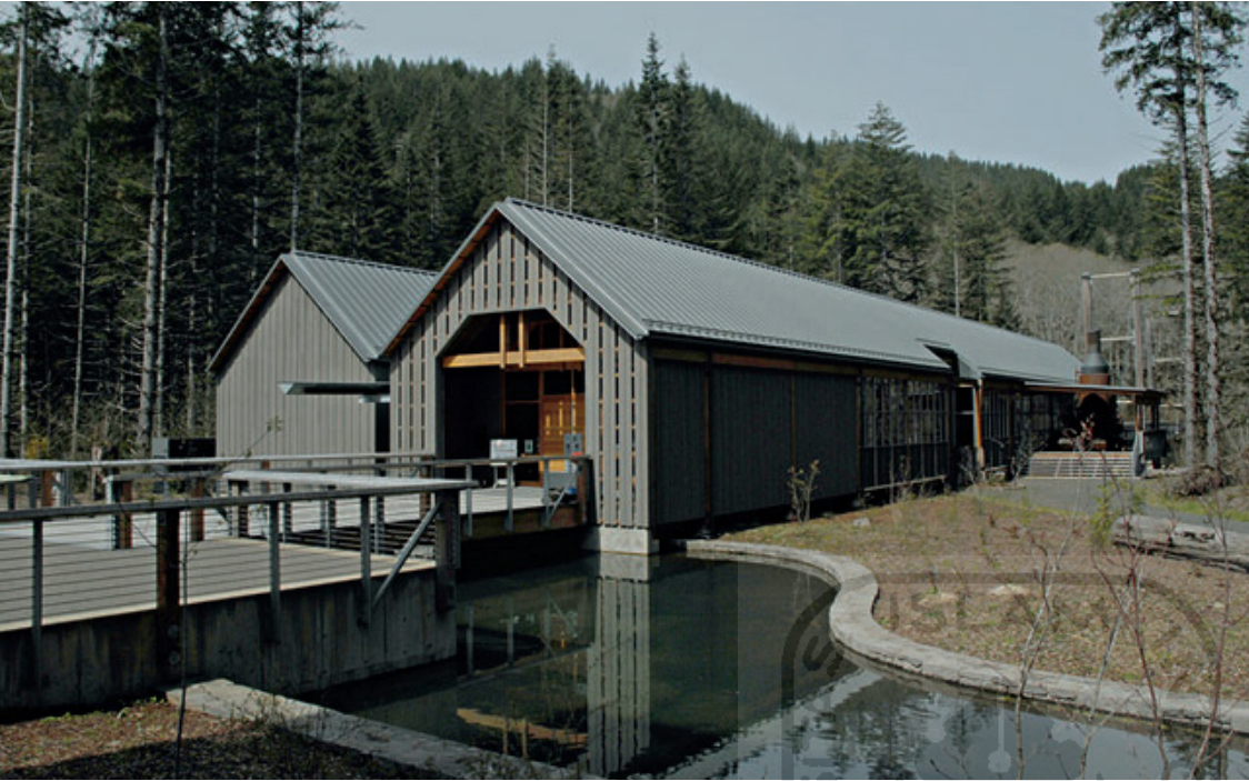
Figure 3.2.13 The 65,000 gallon [246,052 L] forest wetland pond near the entry of the Tillamook Forest Center in Tillamook, Oregon, functions to harvest and store rain water for the fire sprinkler system; provides non-potable water for heat exchange for the cooling system; and serves as a reservoir for structural and wildland fire fighters in the surrounding region.
