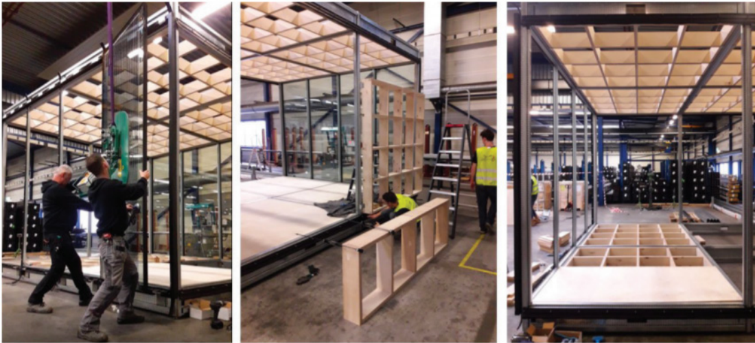
Figure 3.2.10 Illustration of gravity principle of assembly. All parts can be assembled in parallel and create connection only with the main frame. Sources: GTB Lab
