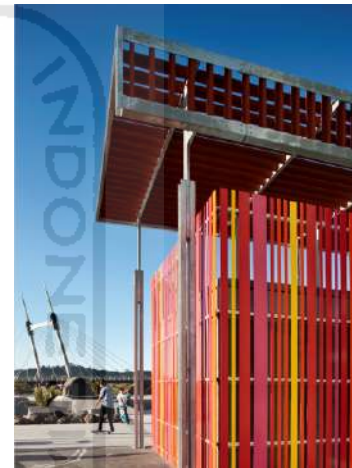
Gambar 47. Fasad Ormiston Activity Centre Sumber : https://www.archdaily.com/
