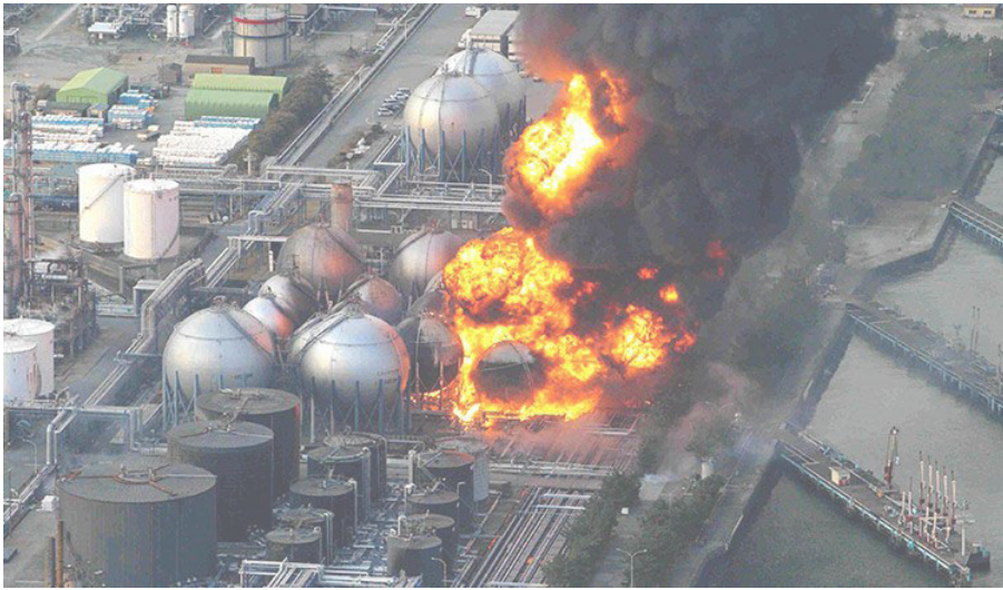
2011 Fukushima nuclear reactor incident, Japan. Source: opensourceinvestigation.com
