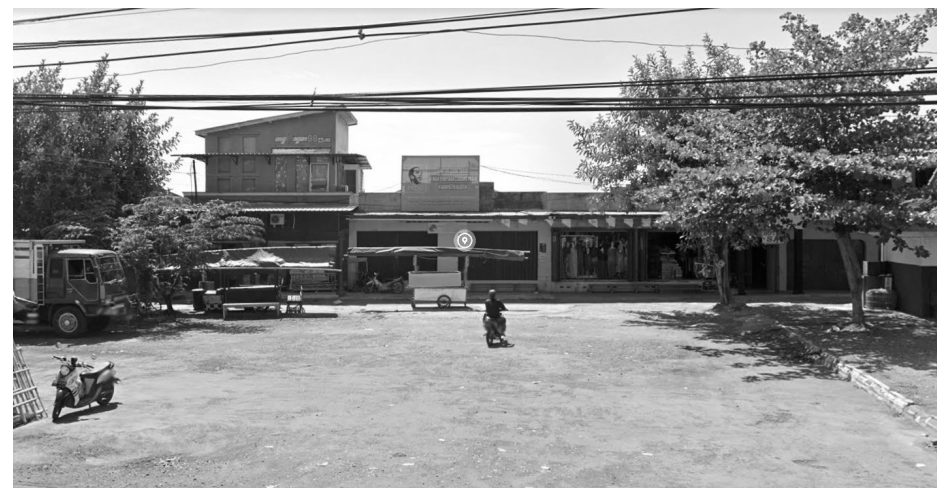
Figure 1.5. Conditions of retail kiosk Source : Google earth
