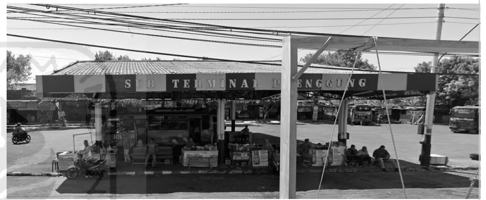
Figure 1.2 Conditions of Penggung bus terminal Source : Google earth
