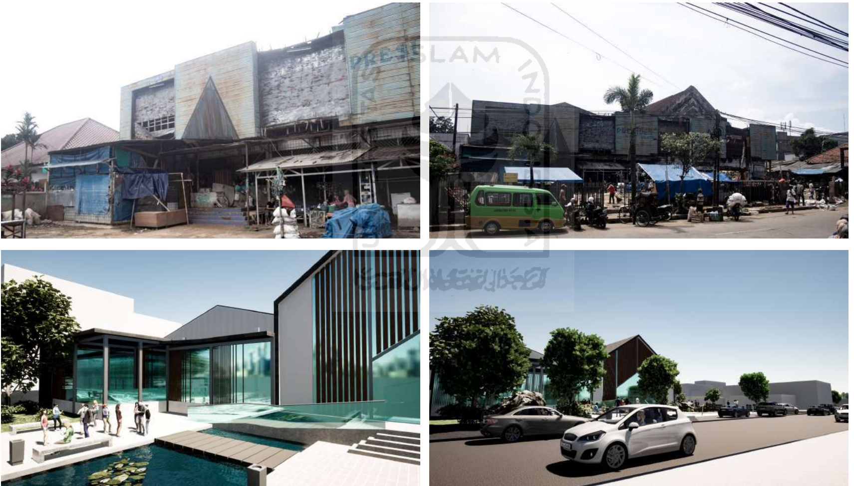
Figure 144: Before and after photo of the facade
