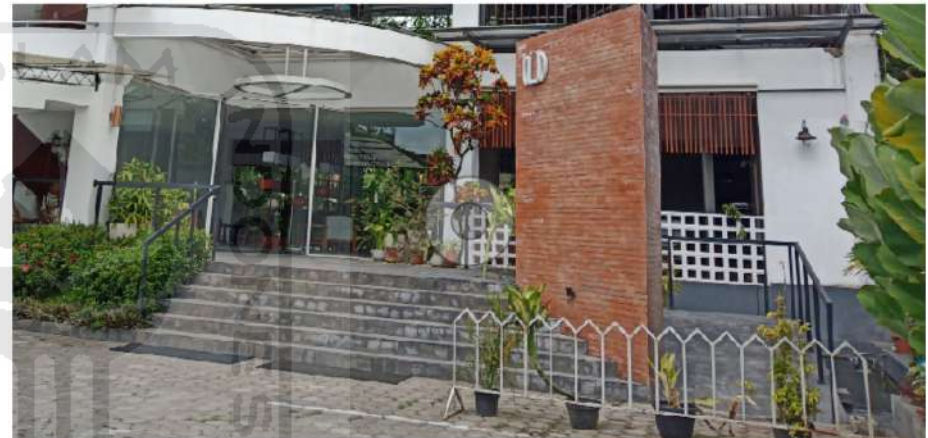
Gambar 4.32 : Entrance Existing Hotel Sumber : Penulis (2019)
