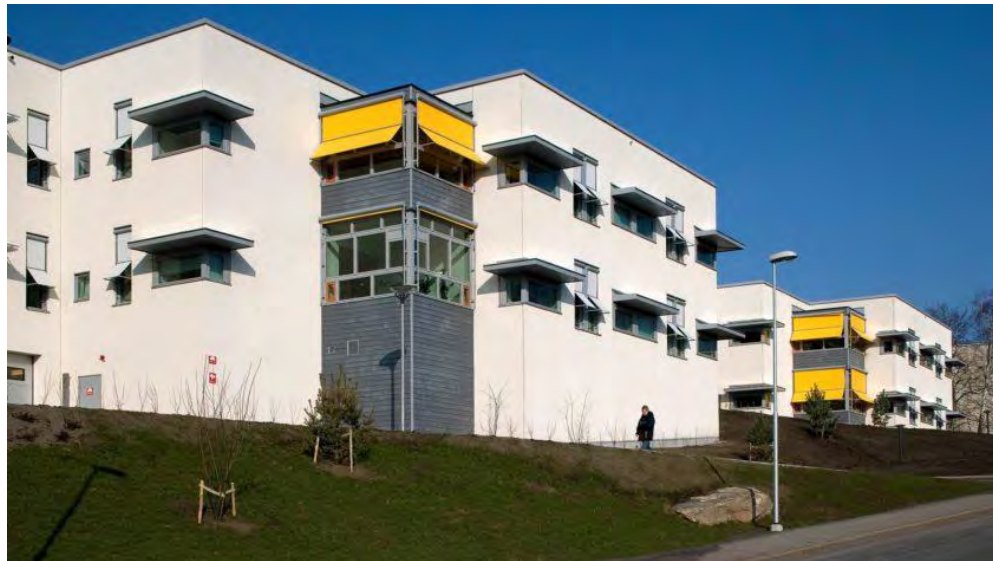
Gambar 2.12 Tampak depan Ostra Hospital Psychiatric Facility
