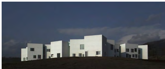
Gambar 2.18 Tampak Depan Children's Center for Psychiatric Rehabilitation
