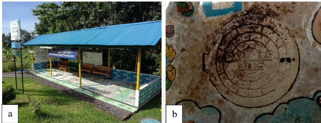
Gambar 7 (a) IPAL Tirto Asri (b) Penutup IPAL
