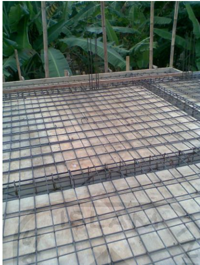
(Gambar 3.10.3 Gambar Atap Cor)
