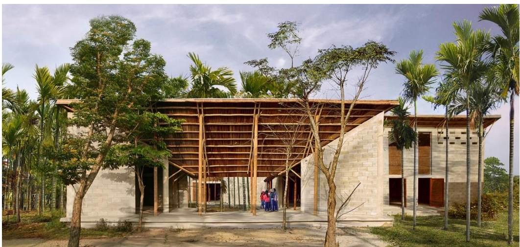
Gambar 2.11 Struktur dan Material Cam Thanh Community ( https://www.archdaily.com/638776/cam-thanh-community-house-1-1-2 , 25/9/2019)
