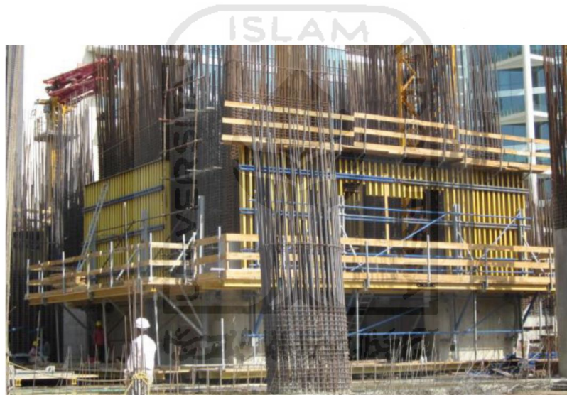
Gambar 3.7 Climbing Formwork System For Lift Core Wall Construction
