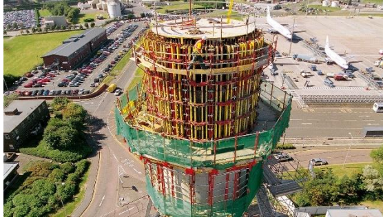
Gambar 5.3 Dinding-Geser tipe bekisting “CB Climbing Formwork”
