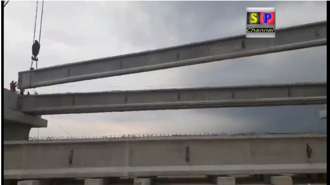
Gambar 5.21. Proses Erection PCI Tol KLBM.
