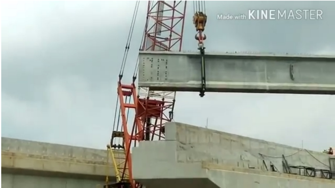
Gambar 5.47. Proses Erection PCI Tol Pantura Gerinsing (Sumber : https://www.youtube.com/watch?v=9tMEC2PnTRc ).
