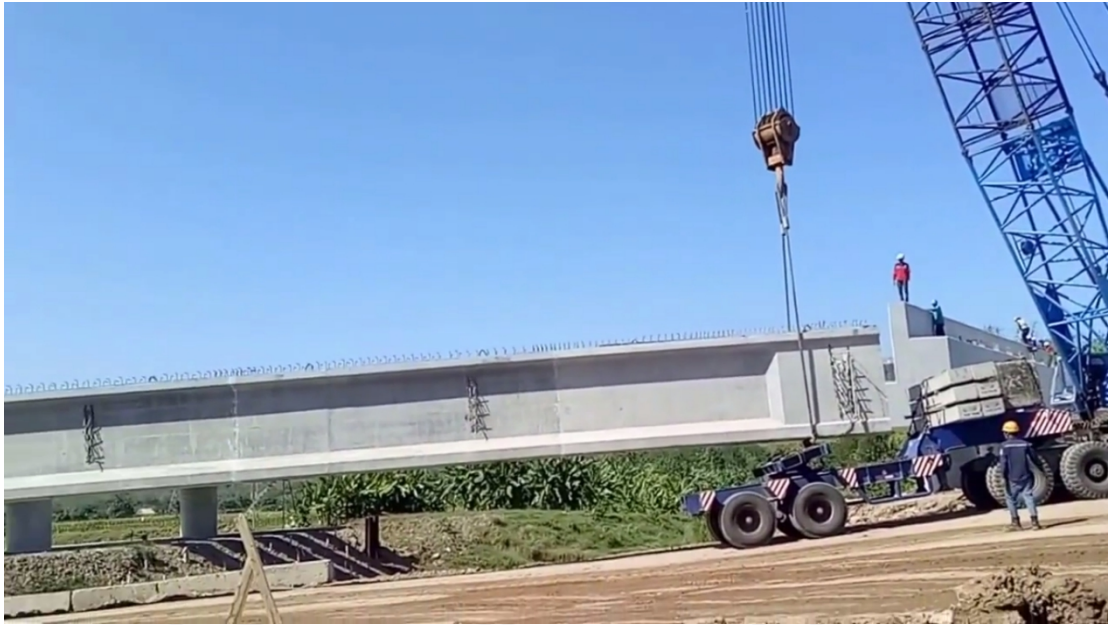
Gambar 5.31. Proses Erection PCI Tol Kendal (Sumber : https://www.youtube.com/watch?v=nFTD9SPzbl4 ).
