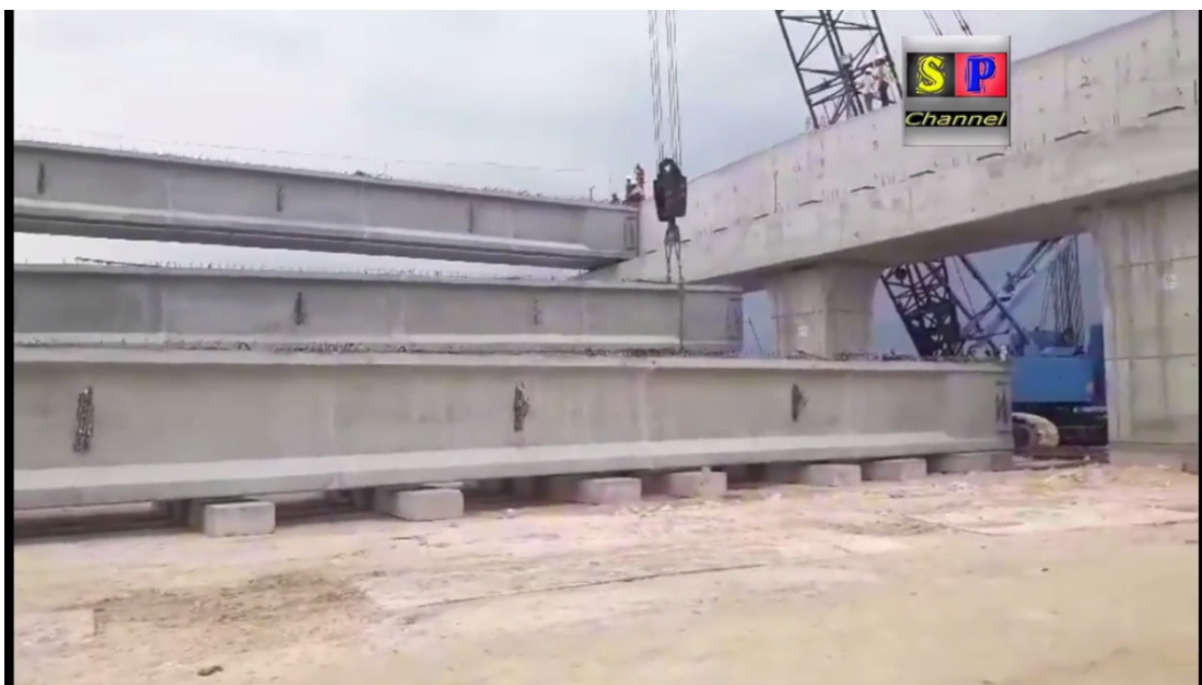
Gambar 5.17. Proses Erection PCI Tol KLBM.
