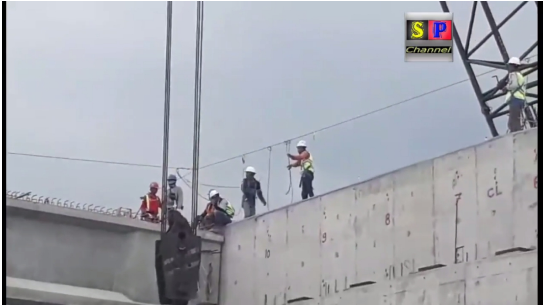
Gambar 5.15. Proses Erection PCI Tol KLBM
