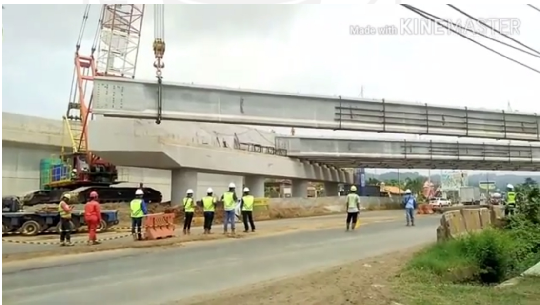
Gambar 5.46. Proses Erection PCI Tol Pantura Geringsing (Sumber : https://www.youtube.com/watch?v=9tMEC2PnTRc ).
