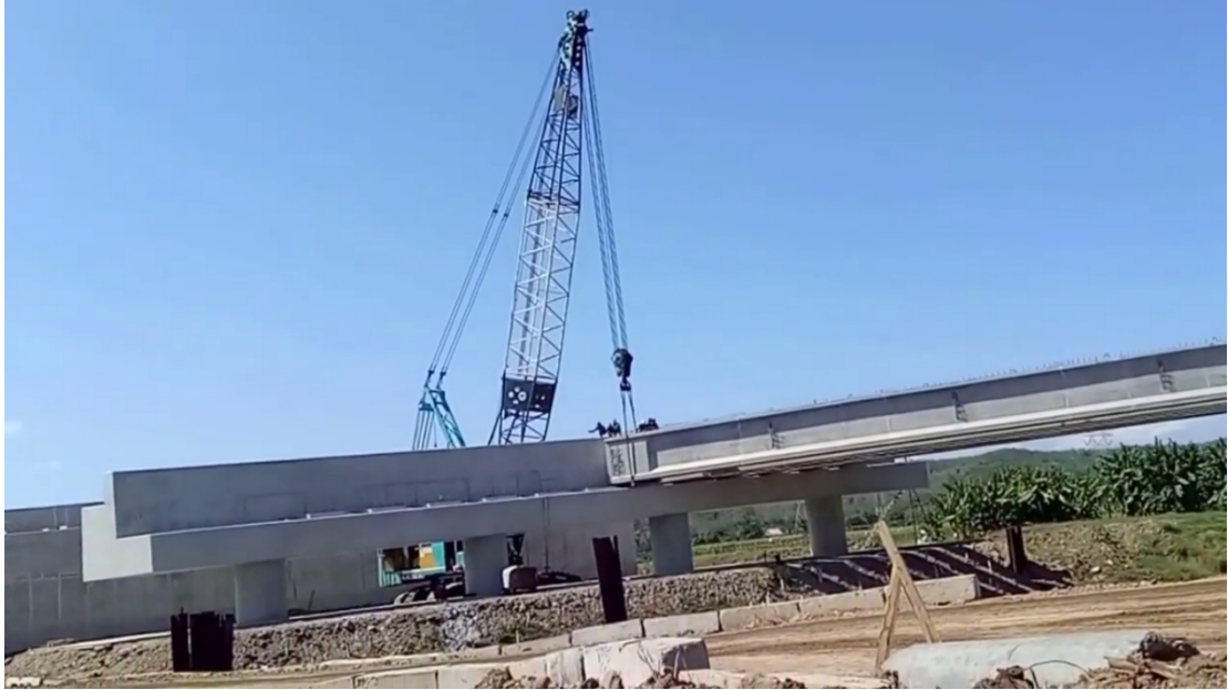
Gambar 5.37. Proses Erection PCI Tol Kendal (Sumber : https://www.youtube.com/watch?v=nFTD9SPzbl4 ).
