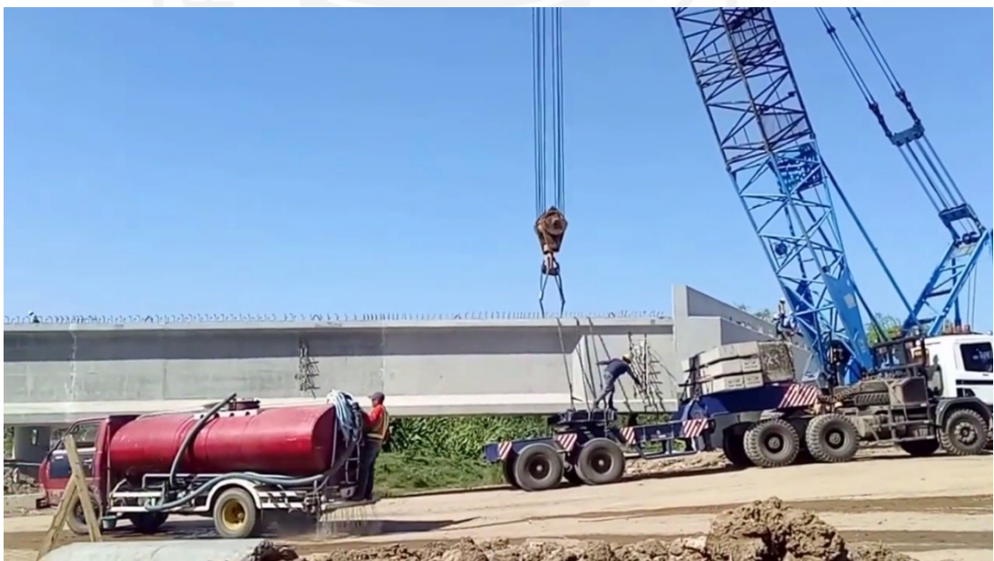
Gambar 5.30. Proses Erection PCI Tol Kendal (Sumber : https://www.youtube.com/watch?v=nFTD9SPzbl4 ).
