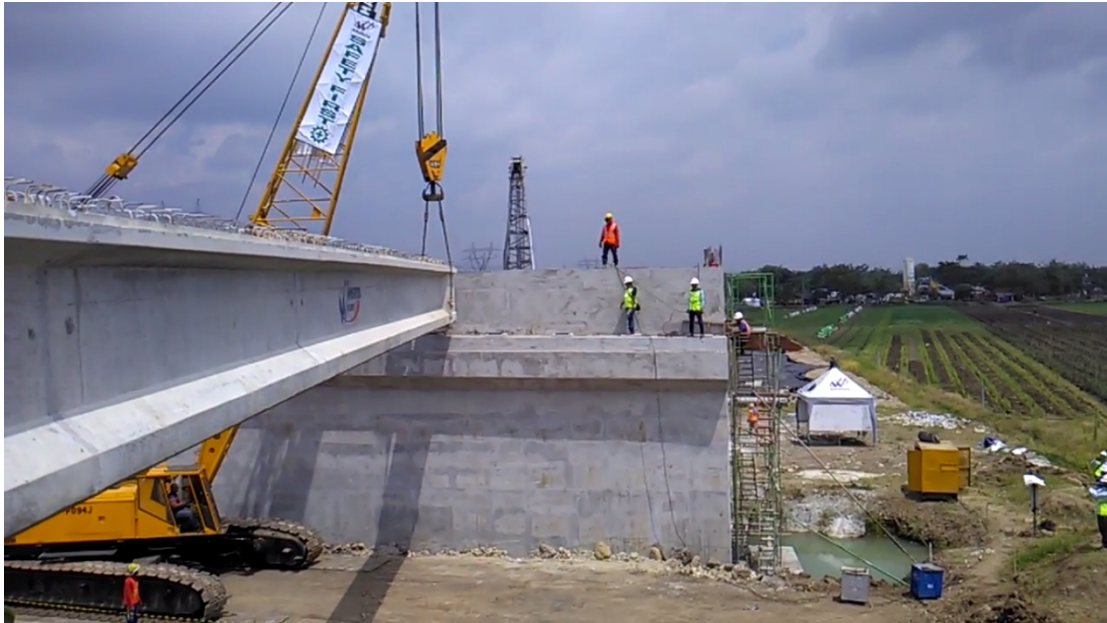
Gambar 5.11. Proses Erection PCI Girder UB Sungai 05 Margomulyo (Sumber : https://www.youtube.com/watch?v=Ny3WqwcxNco&t=383s )
