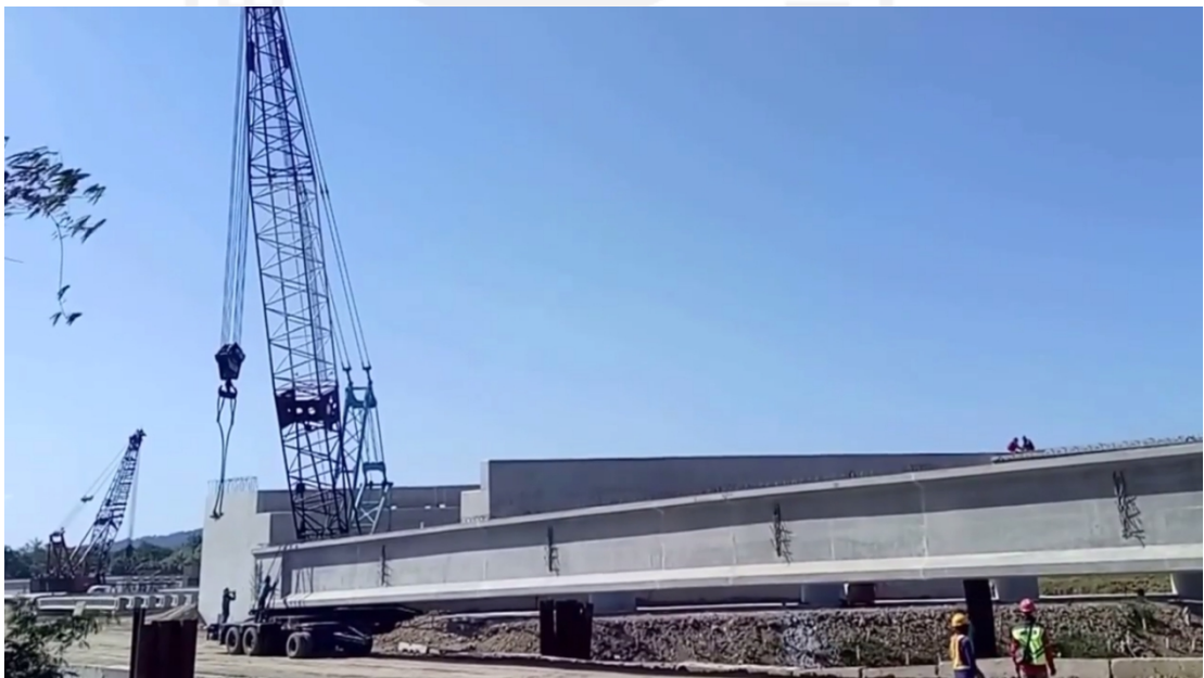
Gambar 5.28. Proses Erection PCI Tol Kendal (Sumber : https://www.youtube.com/watch?v=nFTD9SPzbl4 ).
