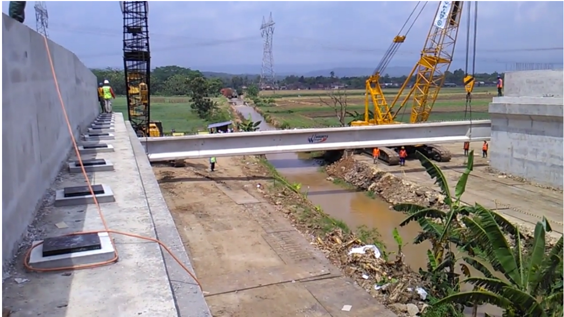
Gambar 5.3. Proses Erection PCI Girder UB Sungai 05 Margomulyo (Sumber : https://www.youtube.com/watch?v=Ny3WqwcxNco&t=383s )
