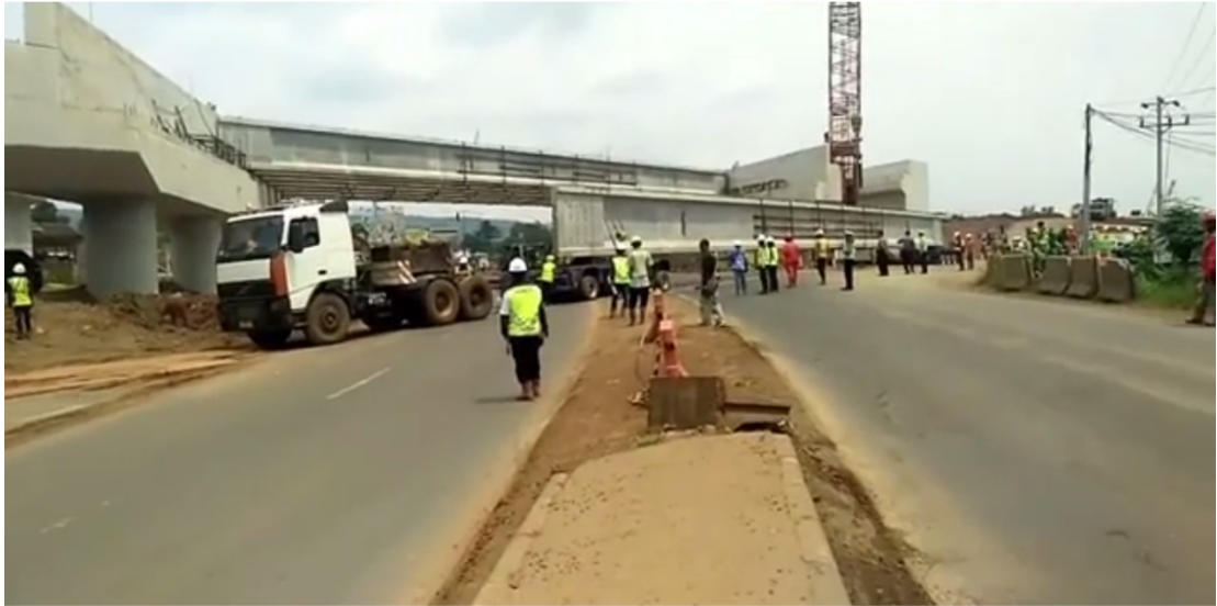
Gambar 5.41. Proses Erection PCI Tol Pantura Gerinsing (Sumber : https://www.youtube.com/watch?v=9tMEC2PnTRc ).
