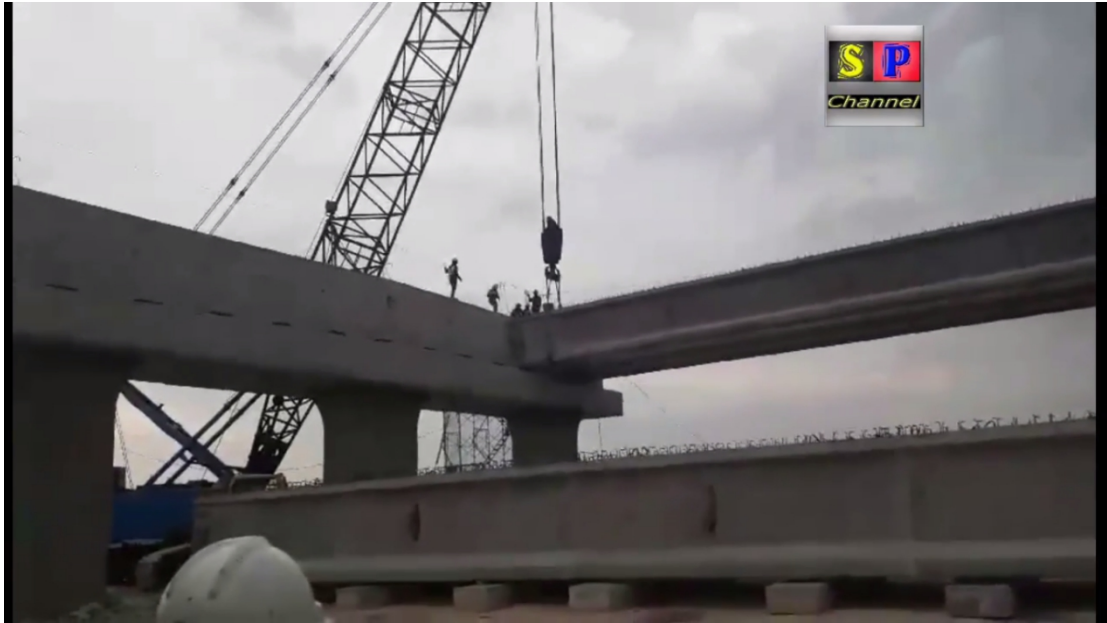
Gambar 5.25. Proses Erection PCI Tol KLBM.
