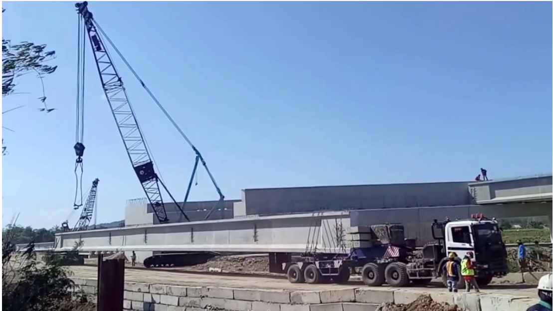
Gambar 5.27. Proses Erection PCI Tol Kendal (Sumber : https://www.youtube.com/watch?v=nFTD9SPzbl4 ).
