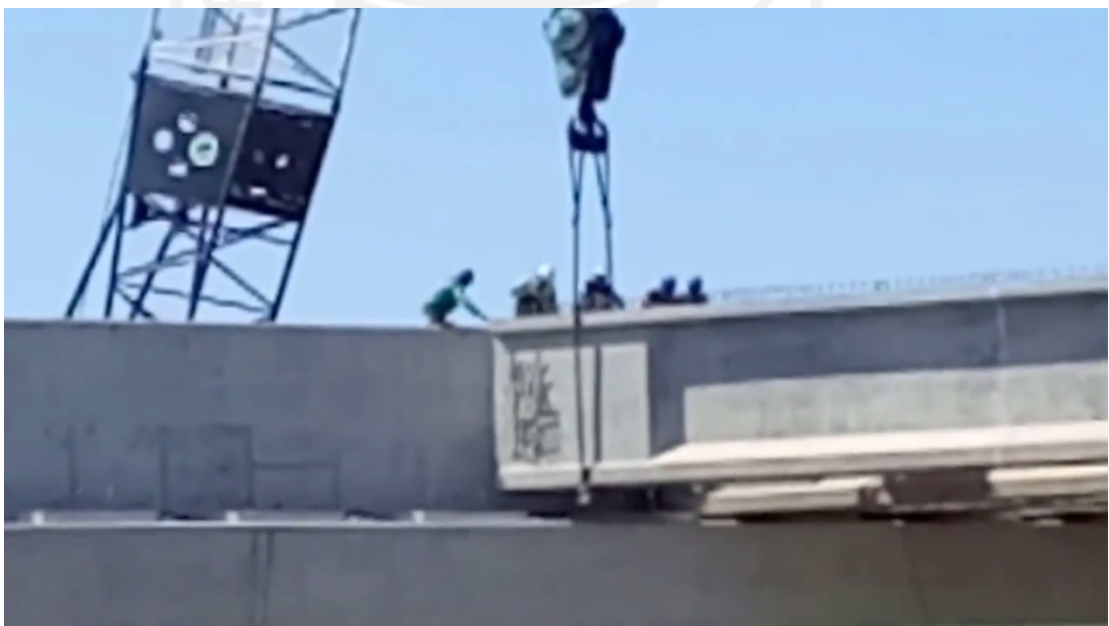
Gambar 5.36. Proses Erection PCI Tol Kendal (Sumber : https://www.youtube.com/watch?v=nFTD9SPzbl4 ).
