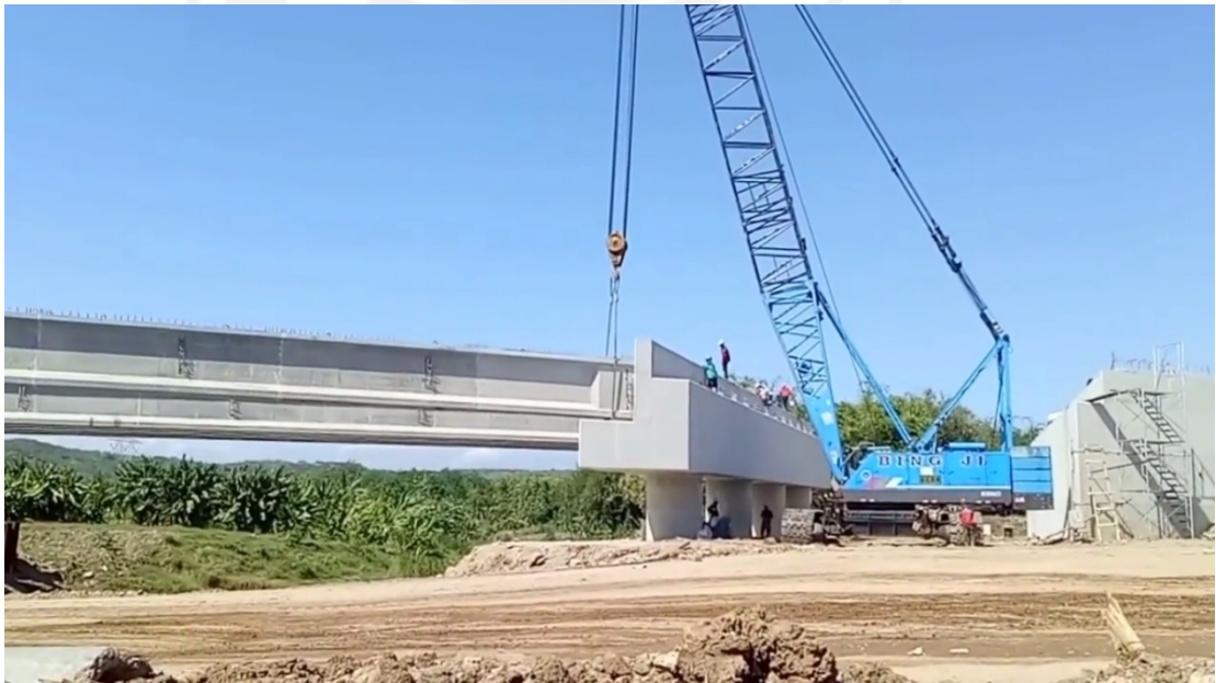
Gambar 5.34. Proses Erection PCI Tol Kendal (Sumber : https://www.youtube.com/watch?v=nFTD9SPzbl4 ).
