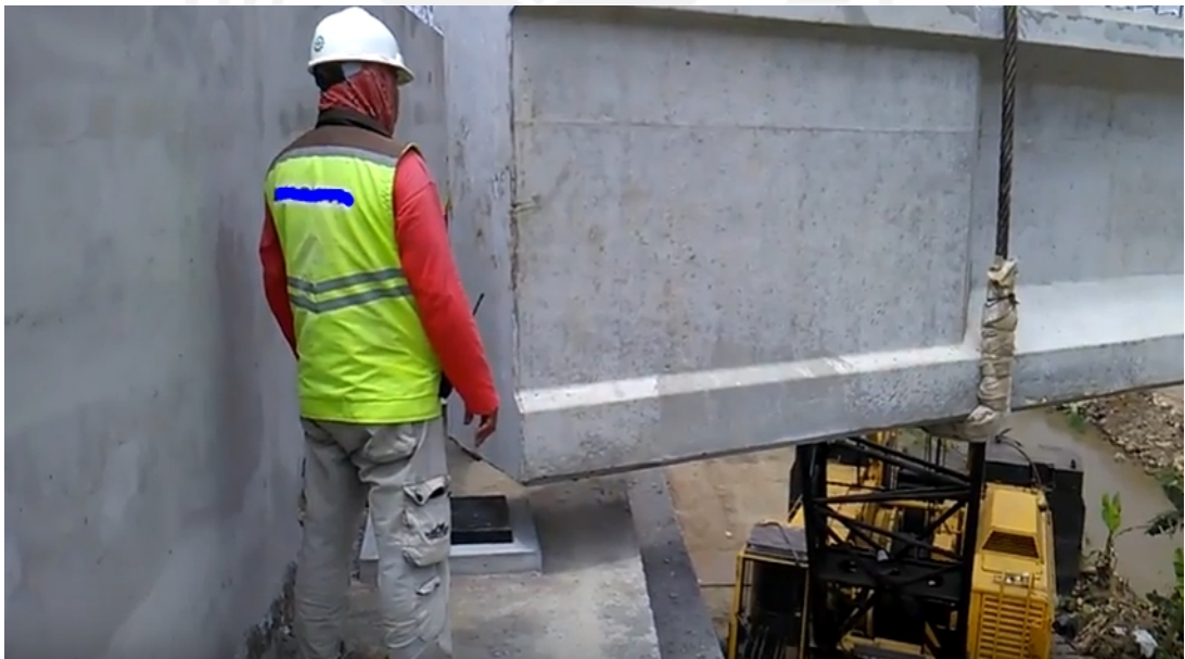
Gambar 5.8. Proses Erection PCI Girder UB Sungai 05 Margomulyo (Sumber : https://www.youtube.com/watch?v=Ny3WqwcxNco&t=383s )
