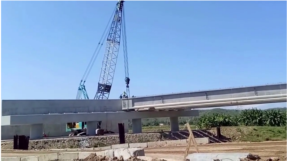
Gambar 5.35. Proses Erection PCI Tol Kendal (Sumber : https://www.youtube.com/watch?v=nFTD9SPzbl4 ).
