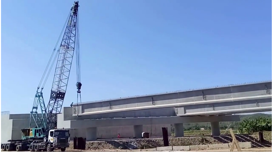
Gambar 5.33. Proses Erection PCI Tol Kendal (Sumber : https://www.youtube.com/watch?v=nFTD9SPzbl4 ).
