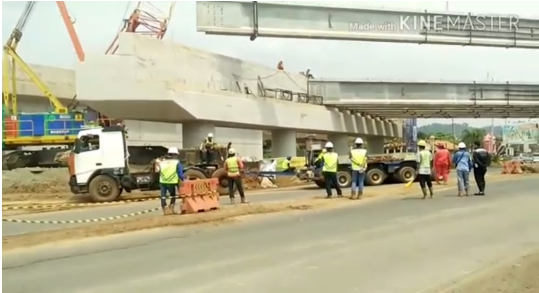
Gambar 5.49. Proses Erection PCI Tol Pantura Geringsing (Sumber : https://www.youtube.com/watch?v=9tMEC2PnTRc ).
