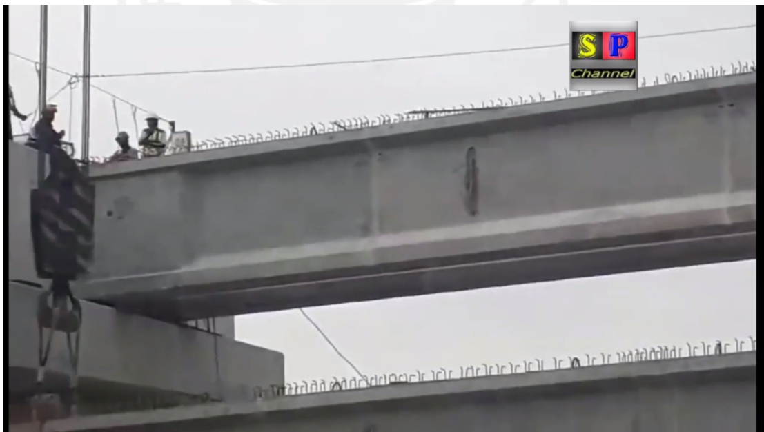
Gambar 5.16. Proses Erection PCI Tol KLBM.
