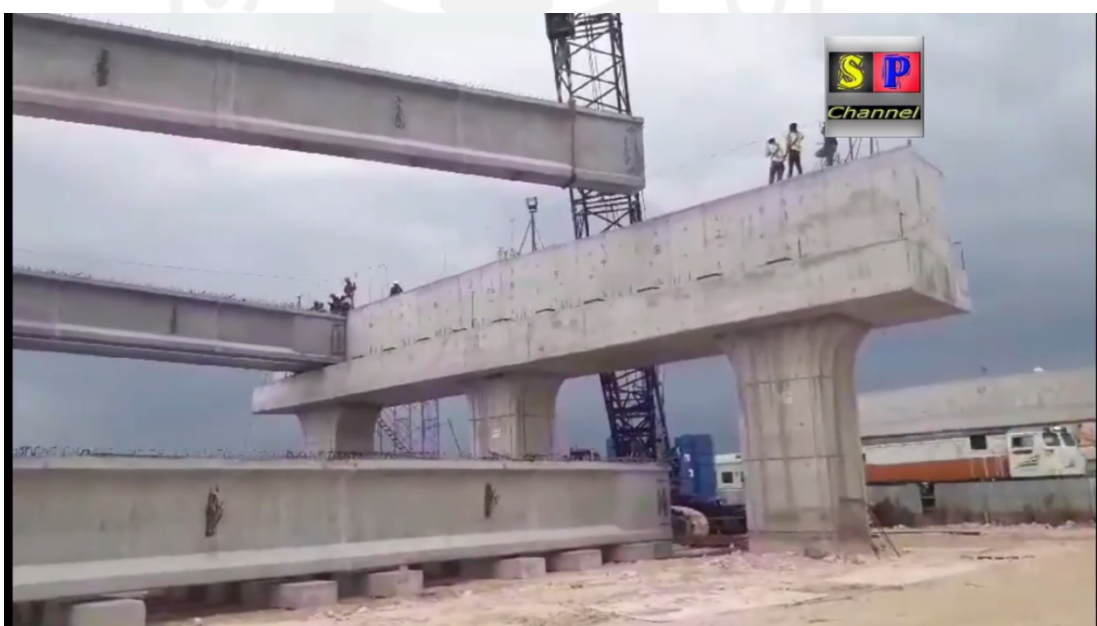
Gambar 5.20. Proses Erection PCI Tol KLBM.
