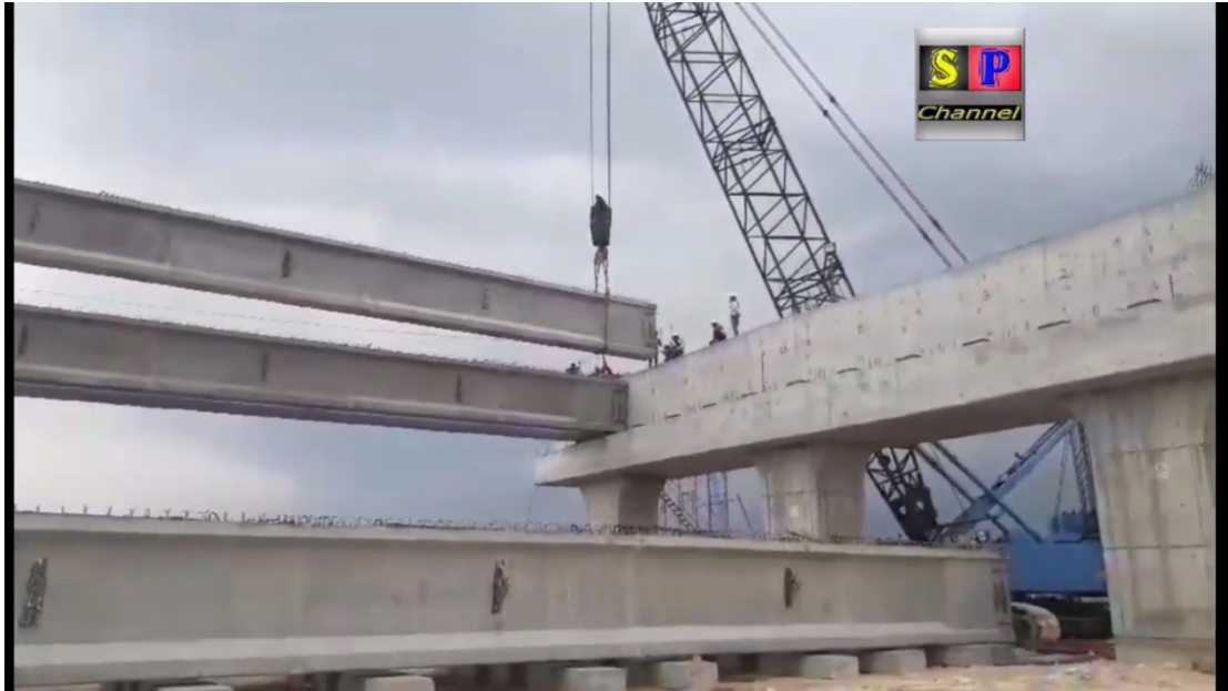
Gambar 5.23. Proses Erection PCI Tol KLBM.
