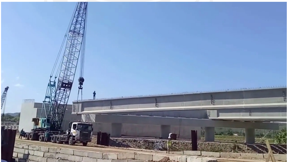
Gambar 5.32. Proses Erection PCI Tol Kendal (Sumber : https://www.youtube.com/watch?v=nFTD9SPzbl4 ).
