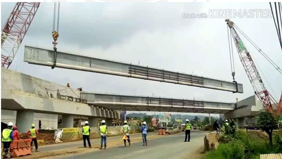
Gambar 5.48. Proses Erection PCI Tol Pantura Gerinsing (Sumber : https://www.youtube.com/watch?v=9tMEC2PnTRc ).
