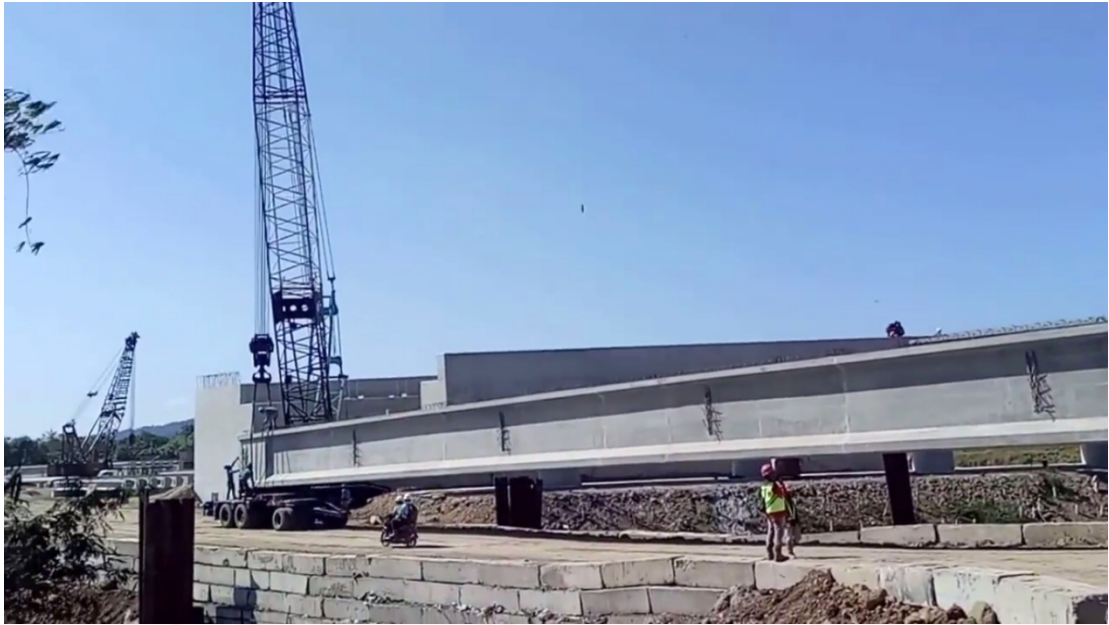
Gambar 5.29. Proses Erection PCI Tol Kendal (Sumber : https://www.youtube.com/watch?v=nFTD9SPzbl4 ).
