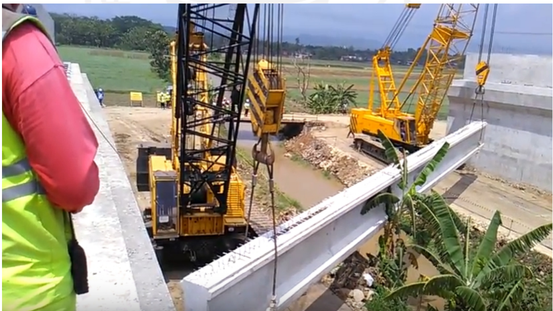
Gambar 5.6. Proses Erection PCI Girder UB Sungai 05 Margomulyo (Sumber : https://www.youtube.com/watch?v=Ny3WqwcxNco&t=383s )
