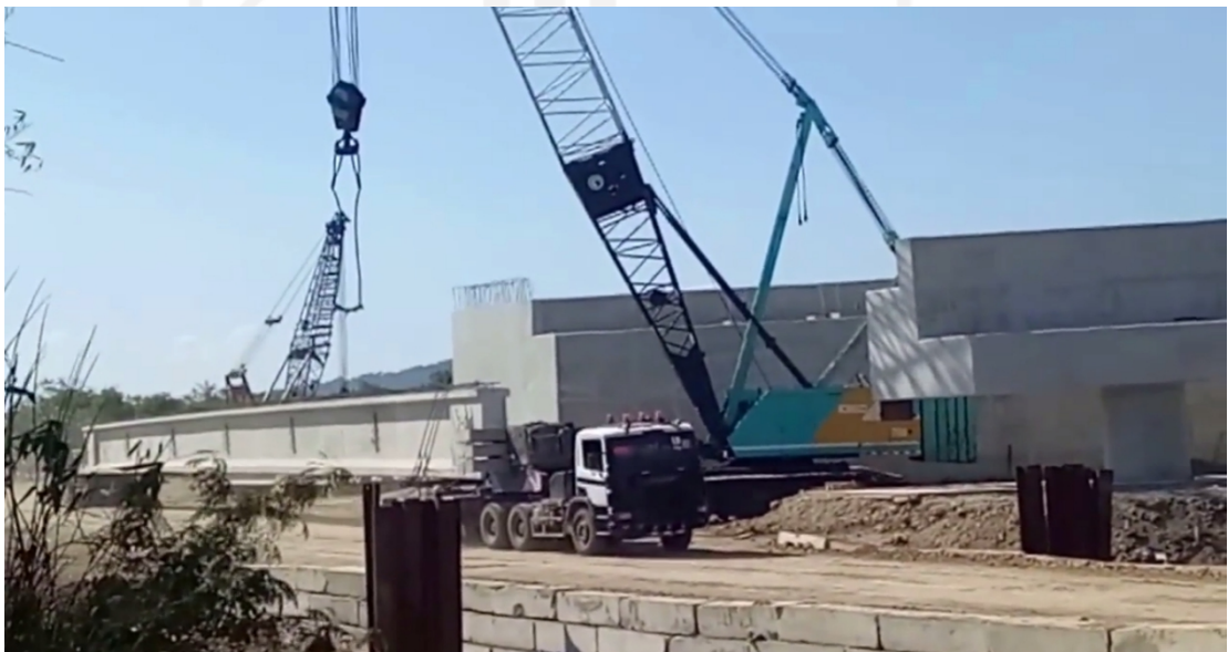
Gambar 5.26. Proses Erection PCI Tol Kendal
