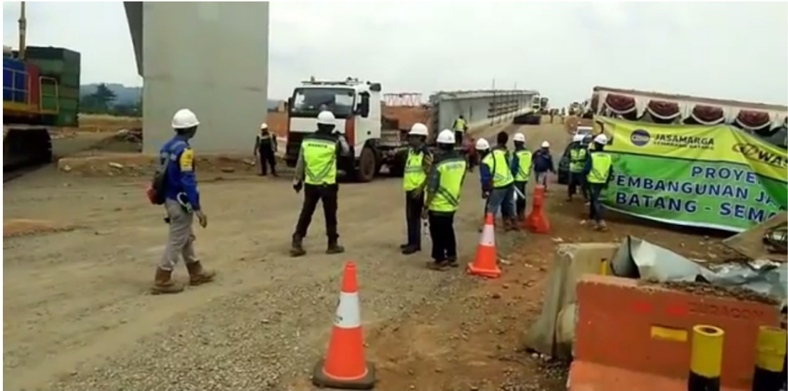
Gambar 5.39. Proses Erection PCI Tol Pantura Geringsing (Sumber : https://www.youtube.com/watch?v=9tMEC2PnTRc ).
