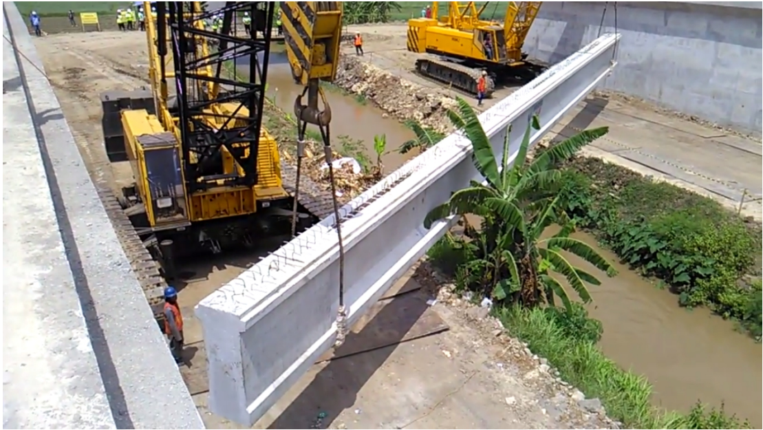
Gambar 5.5. Proses Erection PCI Girder UB Sungai 05 Margomulyo (Sumber : https://www.youtube.com/watch?v=Ny3WqwcxNco&t=383s )
