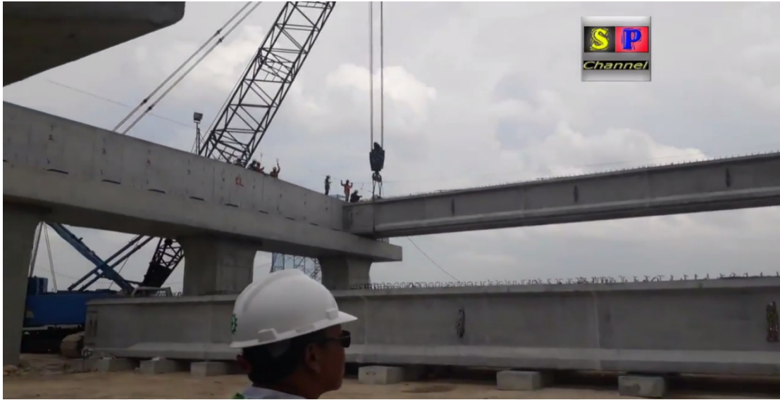
Gambar 5.13. Proses Erection PCI Tol KLBM (Sumber : https://www.youtube.com/watch?v=FLKvgFTMTkM ).
