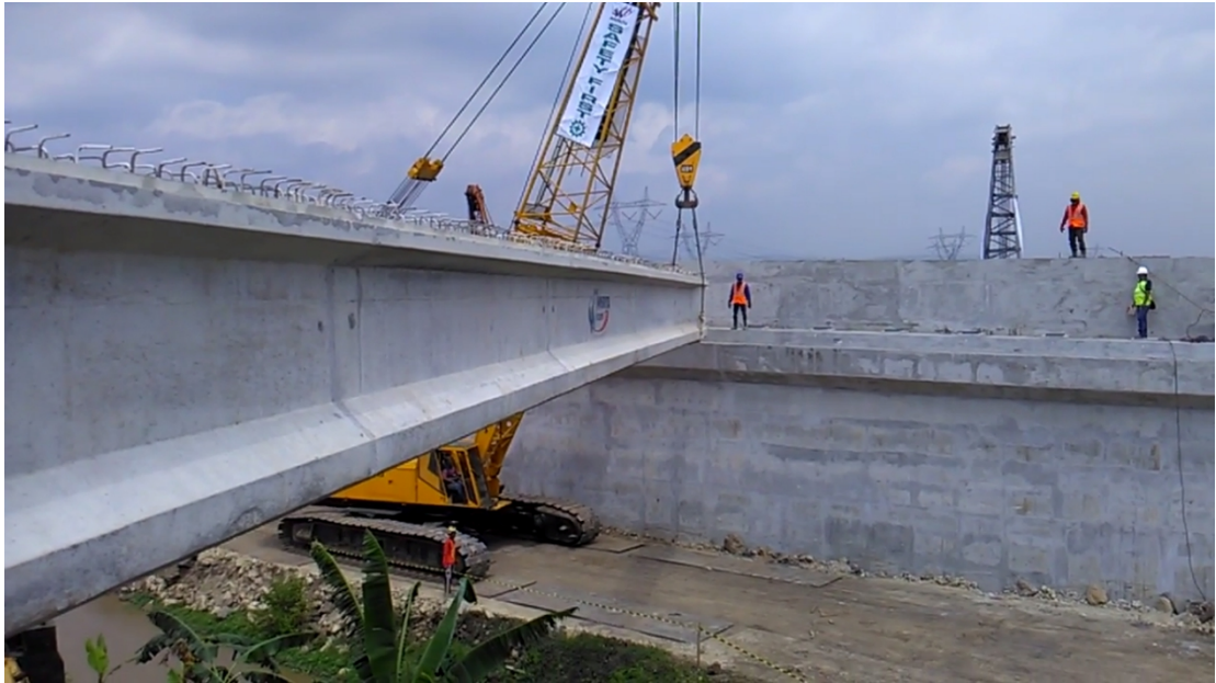
Gambar 5.9. Proses Erection PCI Girder UB Sungai 05 Margomulyo (Sumber : https://www.youtube.com/watch?v=Ny3WqwcxNco&t=383s )
