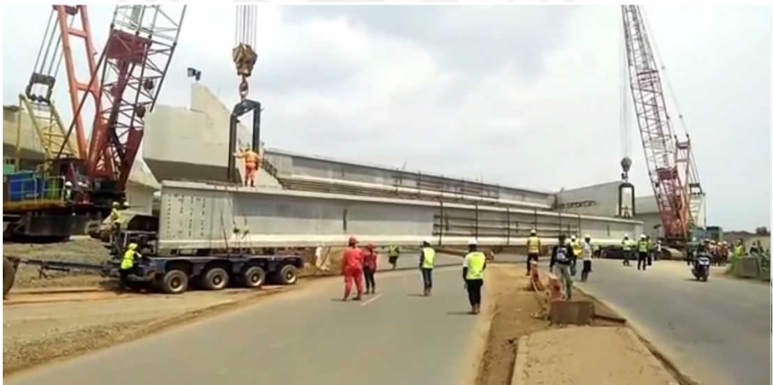
Gambar 5.42. Proses Erection PCI Tol Pantura Gerinsing (Sumber : https://www.youtube.com/watch?v=9tMEC2PnTRc ).
