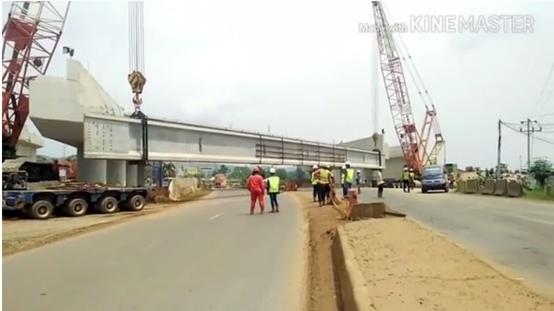
Gambar 5.45. Proses Erection PCI Tol Pantura Geringsing (Sumber : https://www.youtube.com/watch?v=9tMEC2PnTRc ).
