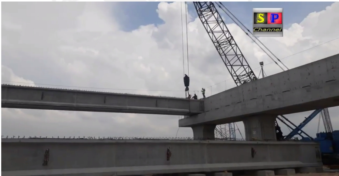
Gambar 5.12. Proses Erection PCI Tol KLBM
