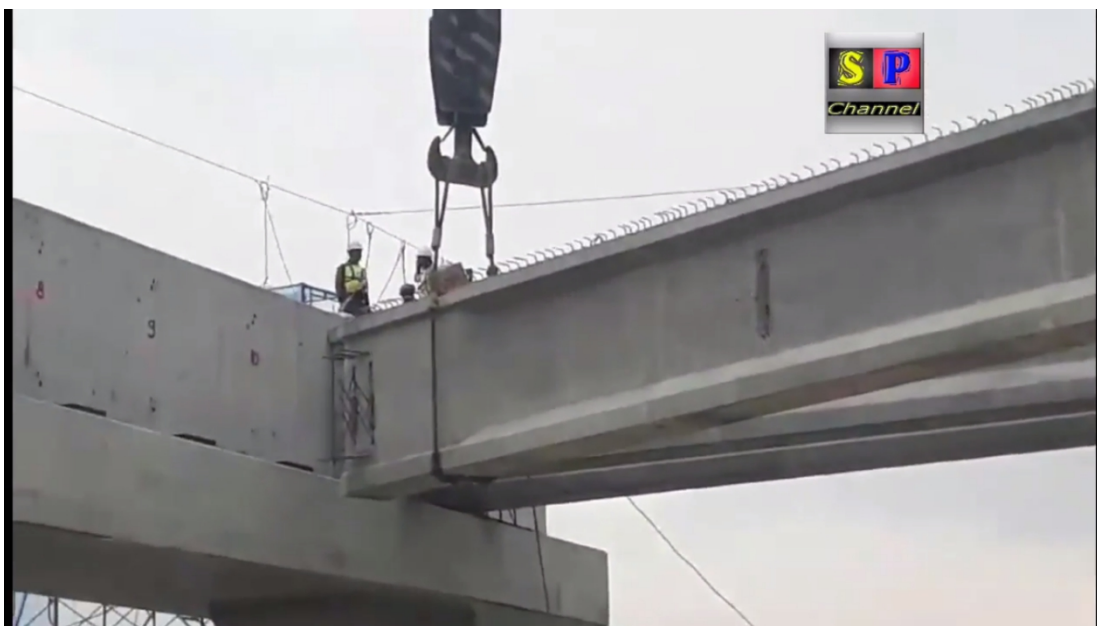
Gambar 5.19. Proses Erection PCI Tol KLBM.
