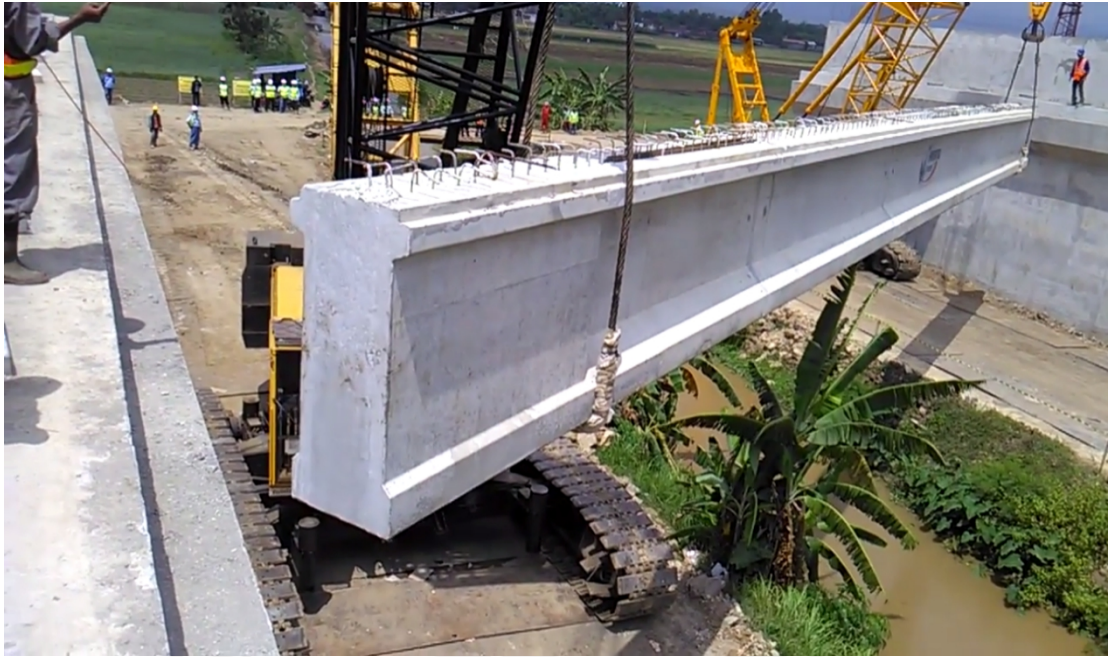
Gambar 5.7. Proses Erection PCI Girder UB Sungai 05 Margomulyo (Sumber : https://www.youtube.com/watch?v=Ny3WqwcxNco&t=383s )
