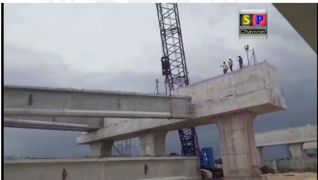
Gambar 5.18. Proses Erection PCI Tol KLBM.
