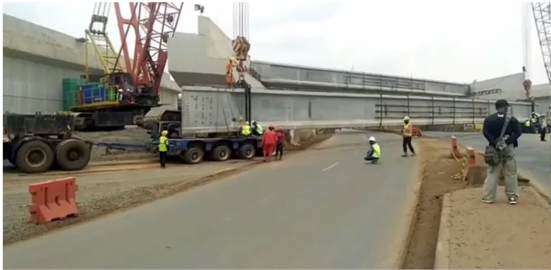
Gambar 5.43. Proses Erection PCI Tol Pantura Geringsing (Sumber : https://www.youtube.com/watch?v=9tMEC2PnTRc ).
