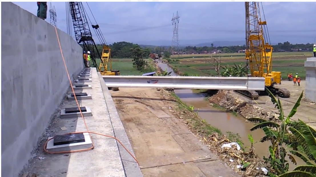
Gambar 5.2. Proses Erection PCI Girder UB Sungai 05 Margomulyo (Sumber : https://www.youtube.com/watch?v=Ny3WqwcxNco&t=383s )
