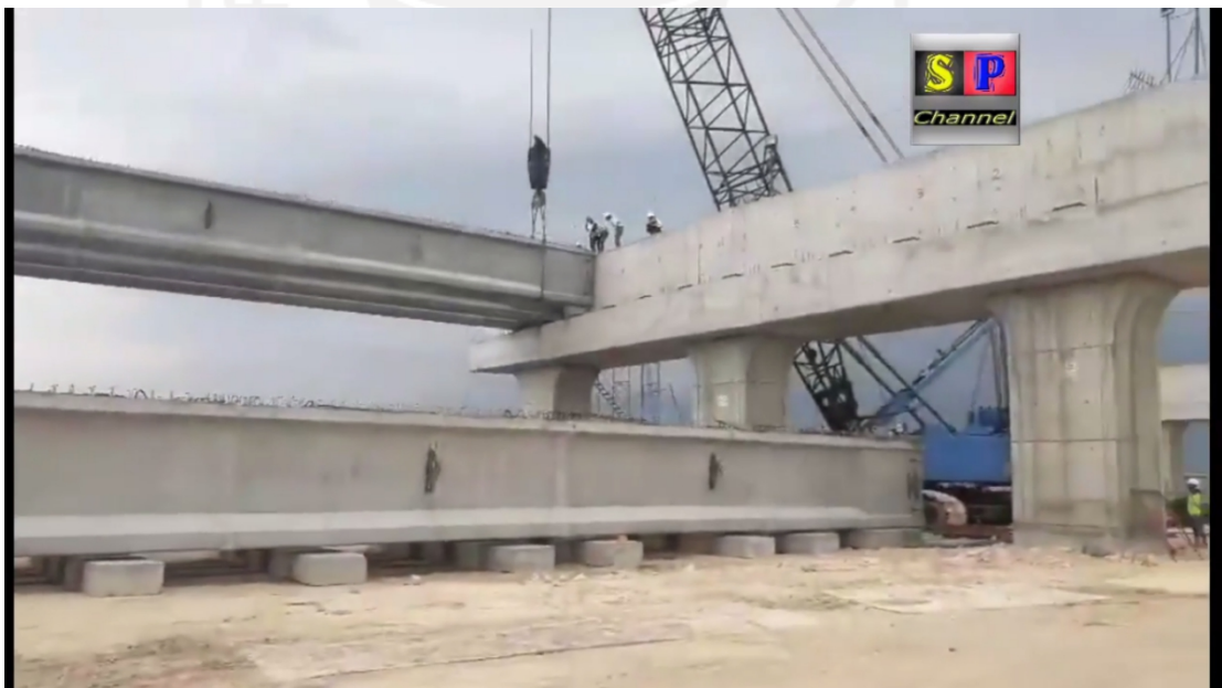
Gambar 5.24. Proses Erection PCI Tol KLBM.
