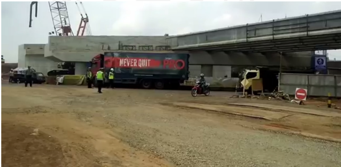
Gambar 5.40. Proses Erection PCI Tol Pantura Geringsing (Sumber : https://www.youtube.com/watch?v=9tMEC2PnTRc ).
