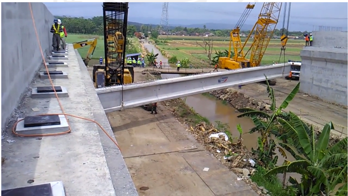
Gambar 5.4. Proses Erection PCI Girder UB Sungai 05 Margomulyo (Sumber : https://www.youtube.com/watch?v=Ny3WqwcxNco&t=383s )
