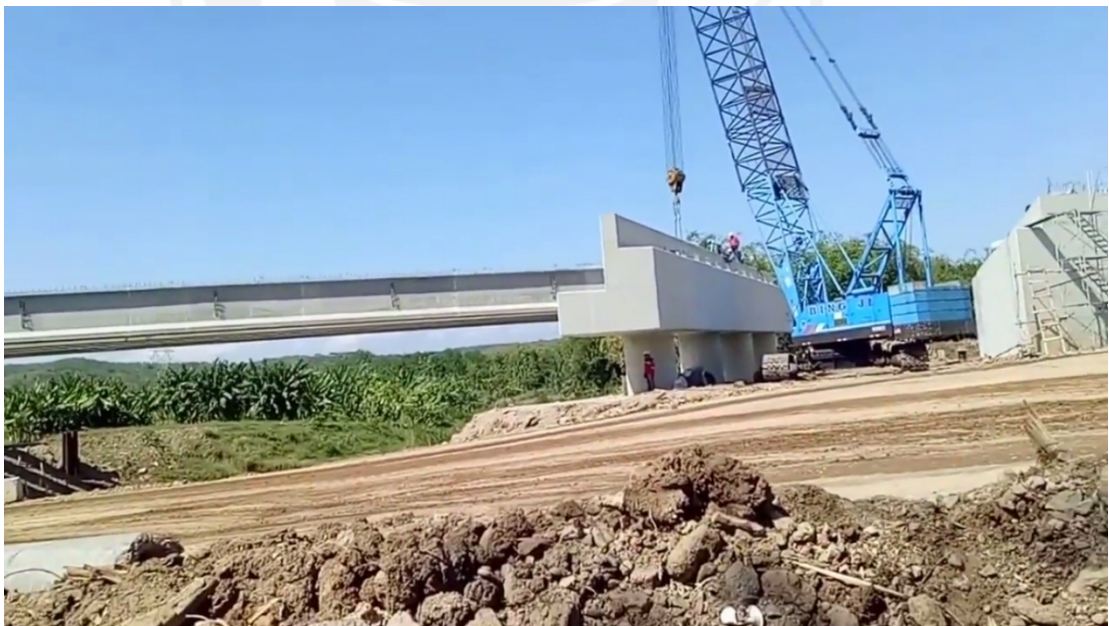
Gambar 5.38. Proses Erection PCI Tol Kendal (Sumber : https://www.youtube.com/watch?v=nFTD9SPzbl4 ).
