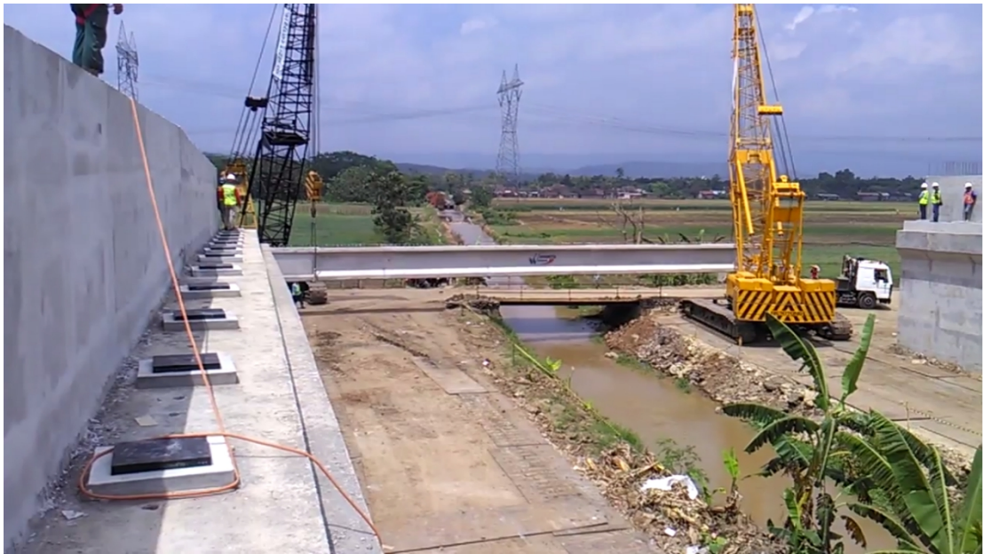
Gambar 5.1. Proses Erection PCI Girder UB Sungai 05 Margomulyo (Sumber : https://www.youtube.com/watch?v=Ny3WqwcxNco&t=383s )
