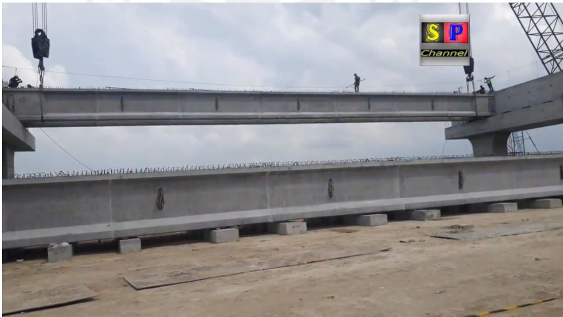
Gambar 5.14. Proses Erection PCI Tol KLBM. (Sumber : https://www.youtube.com/watch?v=FLKvgFTMTkM ).
