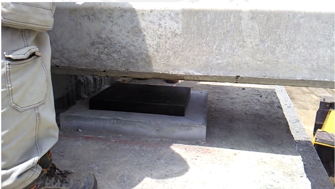
Gambar 5.10. Proses Erection PCI Girder UB Sungai 05 Margomulyo (Sumber : https://www.youtube.com/watch?v=Ny3WqwcxNco&t=383s )
