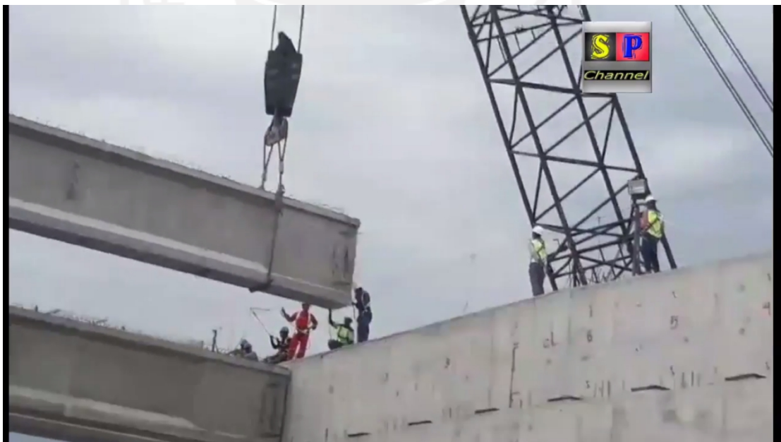
Gambar 5.22. Proses Erection PCI Tol KLBM.
