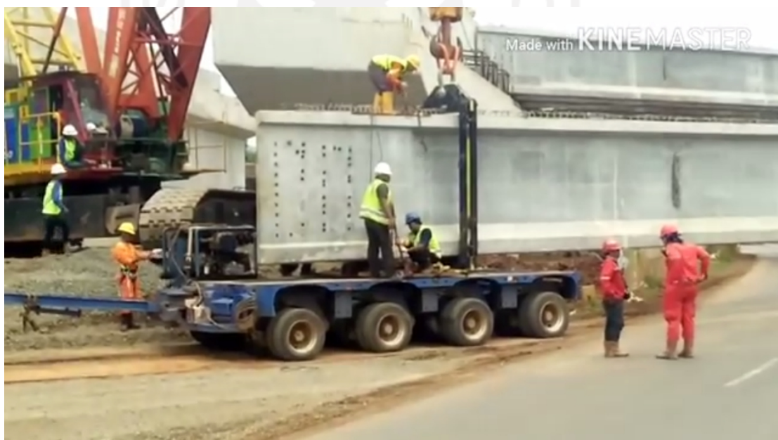
Gambar 5.44. Proses Erection PCI Tol Pantura Geringsing (Sumber : https://www.youtube.com/watch?v=9tMEC2PnTRc ).
