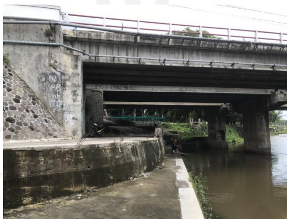
Gambar 5.62 Dinding Penahan Tanah di Depan Abutment
