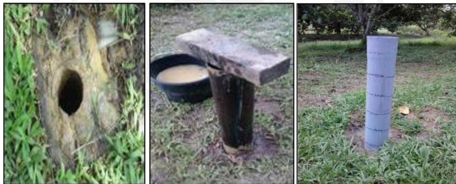
**Gambar 4.39** Lubang Biopori
