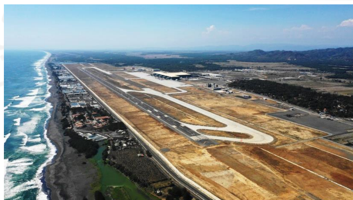
Figure 4.2. An overall view of the airside project
