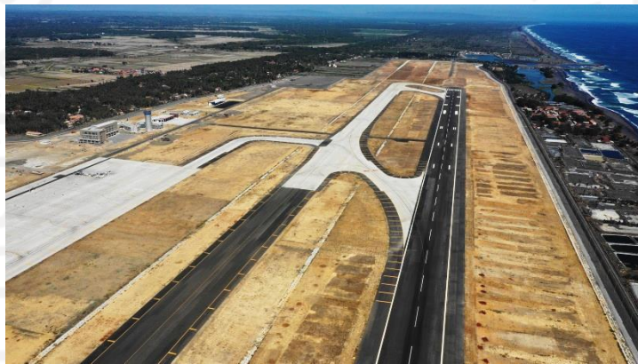
Figure 4.4. Top view of the pavement runway work
