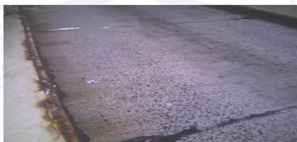
Gambar 3.35 Pelepasan Pengausan ( Polished Aggregate )
