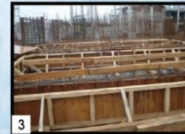
3 Letakkan Union Floor Deck W-1000® di atas penyangga sementara Place Union Floor Deck W-1000® above temporary support
