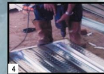
4 Endstop metal dipasang pada Union Floor Deck W-1000® Install the metal endstop to Union Floor Deck W-1000®
