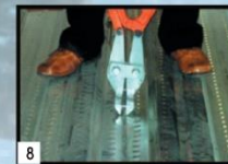
8 Sambungan Union Floor Deck W-1000® dapat diperkaku dengan jepitan Union Floor Deck W-1000® joint can be strengthened by pinching
