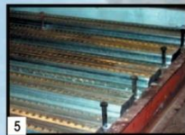
5 Pasang penghubung geser Install the shear connector
