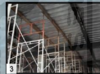
3 Letakkan Union Floor Deck W-1000® di atas penyangga sementara Place Union Floor Deck W-1000® above temporary support
