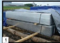
1 Buka bundel Union Floor Deck W-1000® Unfasten the bundle of Union Floor Deck W-1000®
