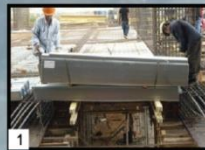
1 Buka bundel Union Floor Deck W-1000® Unfasten the bundle of Union Floor Deck W-1000®
