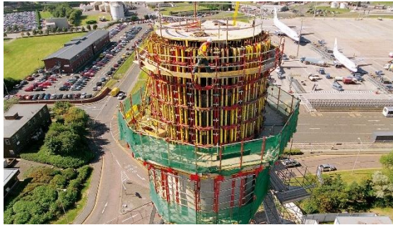
Gambar 5.3 Dinding-Geser tipe bekisting “CB Climbing Formwork”
