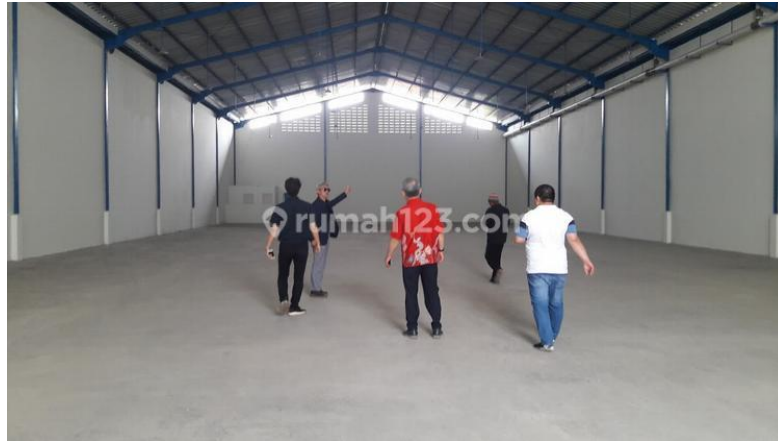
Figure 4.4 Inside look Warehouse B
