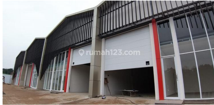
Figure 4.1 Outside look of Warehouse A
