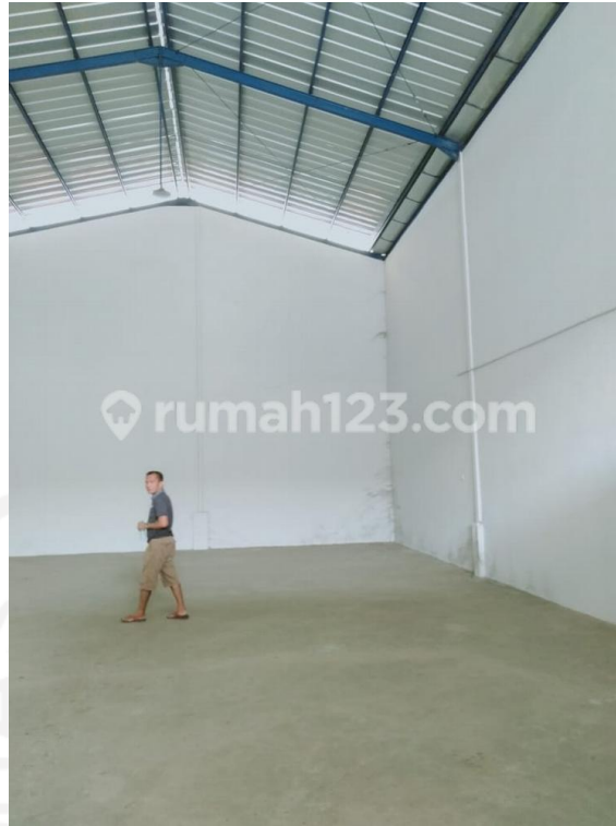
Figure 4.6 Inside look Warehouse C
