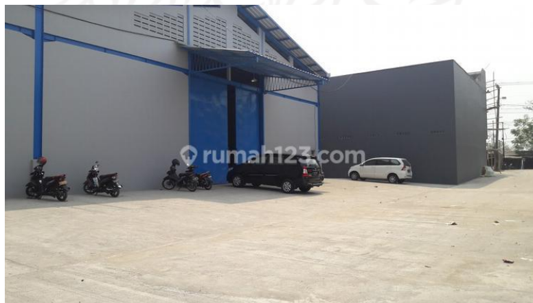
Figure 4.3 Outside look Warehouse B
