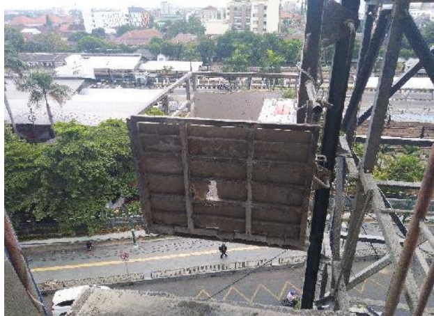
Gambar 3. 17 Material Hoist
