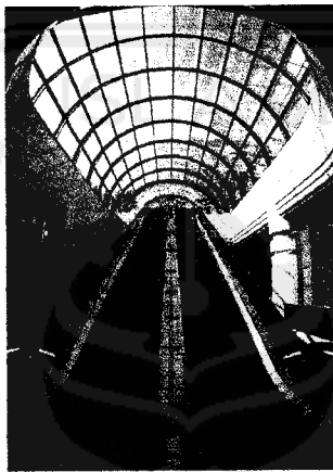
Gambar 136. Transportasi vertical Eskalator
