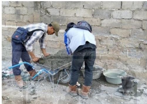
Gambar 5.16 Proses Pengendalian Mutu Beton
