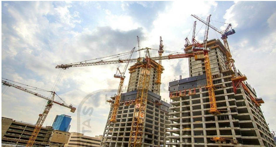
Gambar 3.3 Climbing Tower Crane (Sumber: Sky-line.co.il)
