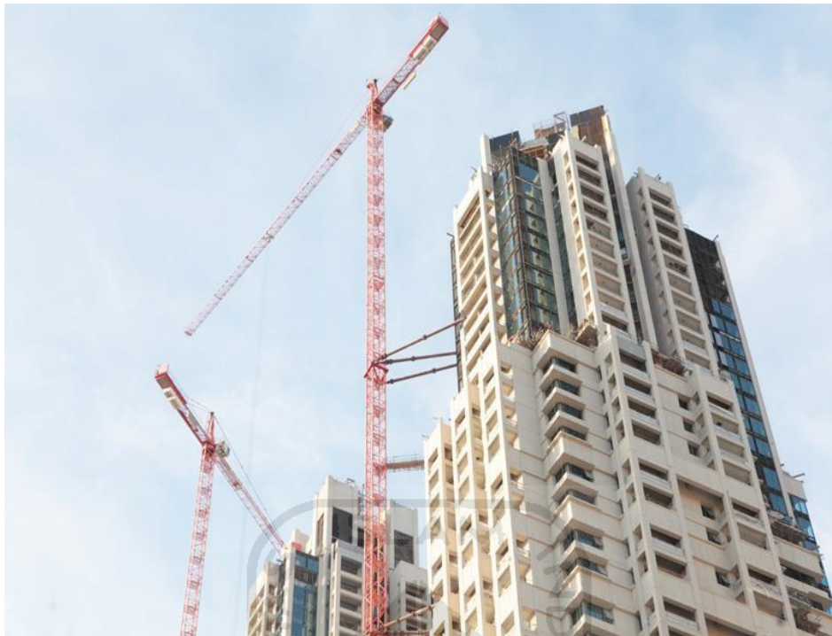
Gambar 3.4 Tied In Crane
