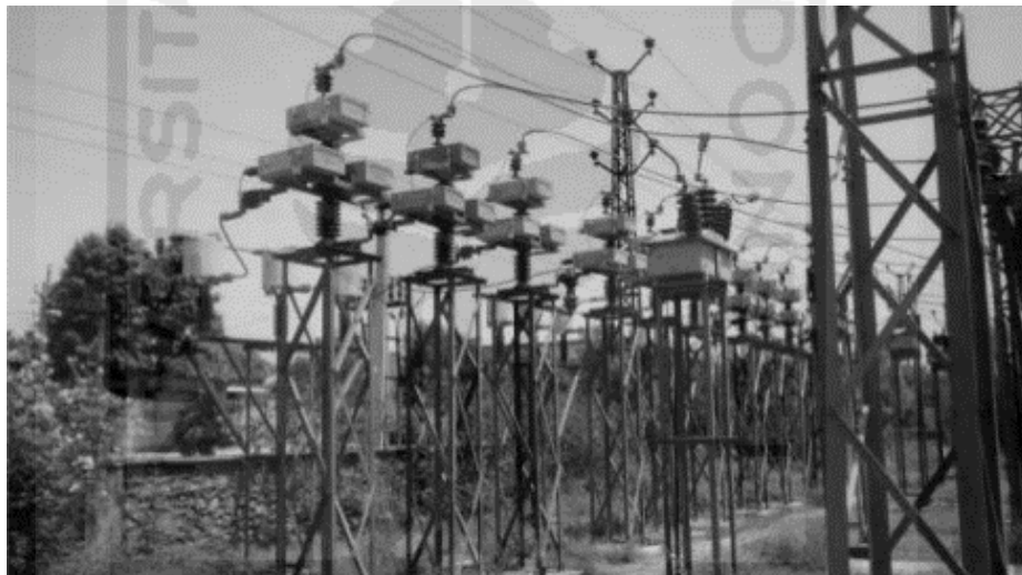
Gambar 2.2 Capacitor Bank
