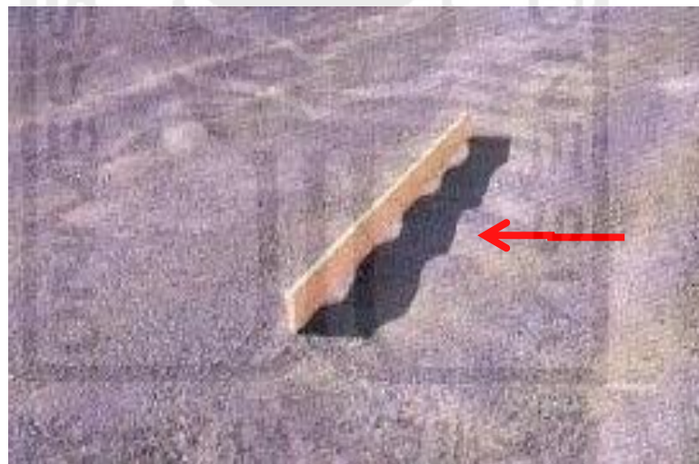
Gambar 3.4 Keriting ( Corrugation ) (Sumber : Bahlawant, 2011)
