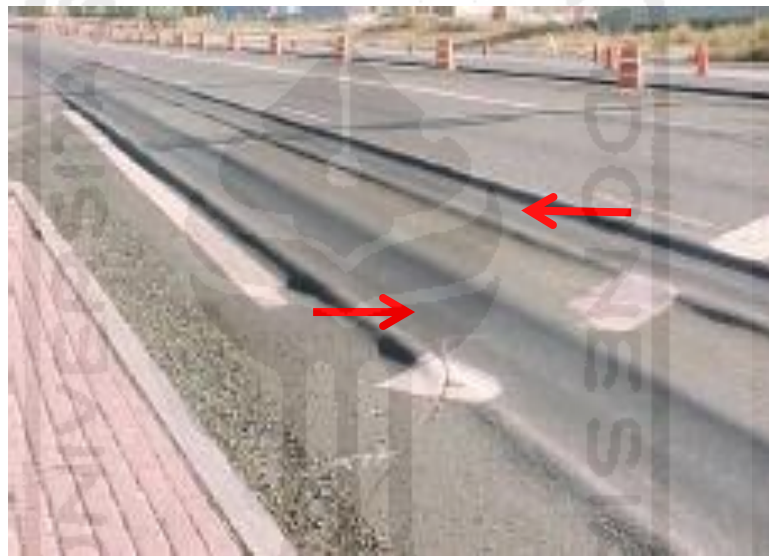
Gambar 3.11 Alur ( Rutting ) (Sumber : Hafid, 2013)
