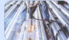
Step 6 Fix SMARTDEK™ to steel or concrete beam if required
