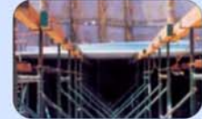
Step 2 Place temporary support if required
