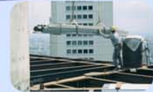
Step 1 Open SMARTDEK™ sheet bundles
