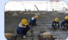
Step 8 Place reinforcement
