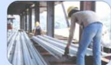
Step 4 Place on steel or concrete beam
