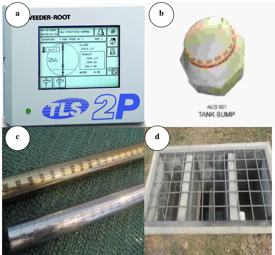
Gambar 4.8 Fasilitas Pendukung SPBU (a) Automatic Tank Gauging, (b) Tank Sump, (c) Stick (tongkat duga), (d) Oil catcher
