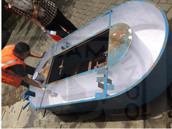
Gambar 2 Persiapan reaktor oxidation ditch
