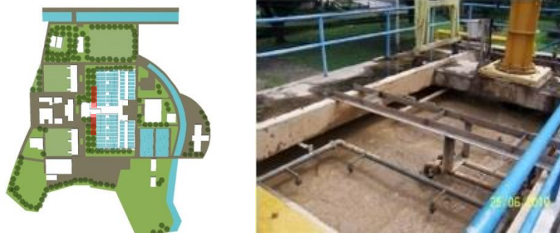
Gambar 2.17 Bangunan Mixing Basin
