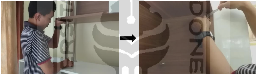
Gambar 4-25 Proses Pemasangan Stainless Steel
