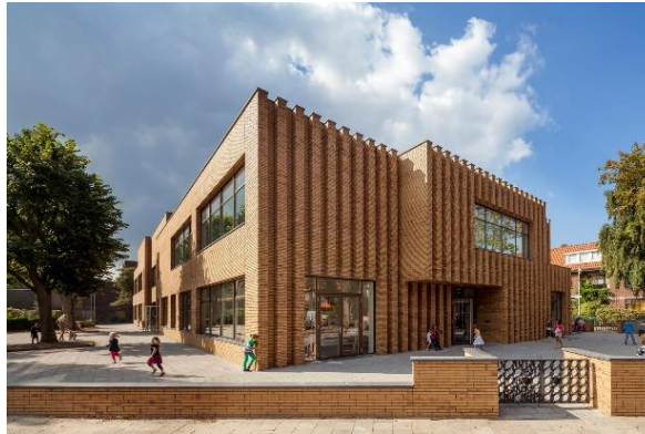
Gambar 2.37 Montessori School Waalsdorp
