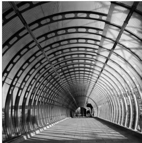
Gambar 2.6.3 Curved steel support for walkway enclosure
