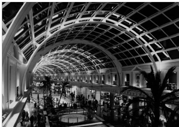
Gambar 2.6.1 Curved roof steelwork to retail center
