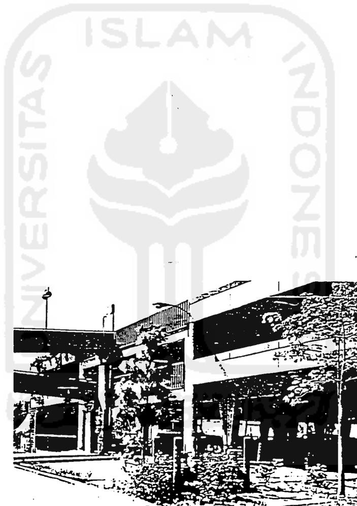
3-31 This parking structure combines precast and poured-in-place concrete construction. Pedestrian skyways lead to the retail portion of the complex.
