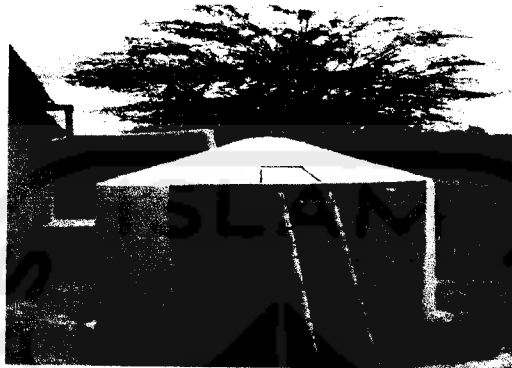
Gambar 3. wire-mesh concrete cistern 10 000 l Sumber : Gnadlinger Johann , 1997
