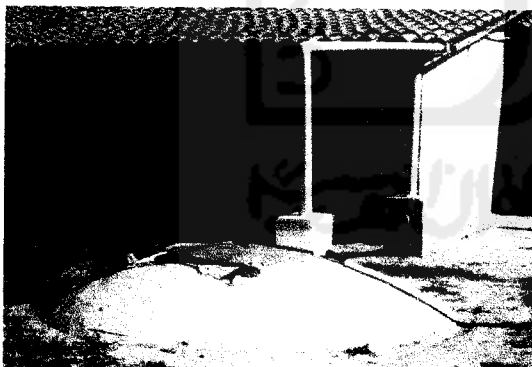
Gambar 4. Underground lime and bricks cistern Sumber : Gnadlinger Johann, 1997
