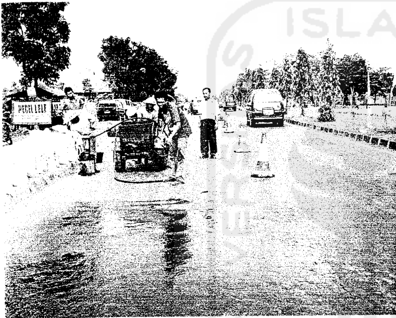
Disiram aspal dg. Asphalt Sprayer
