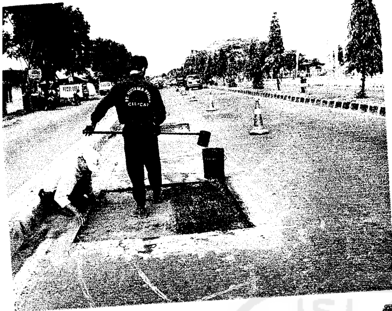
Disiram aspal dg. canting
