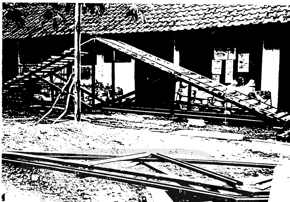
Gambar 1. Rangka Howe
