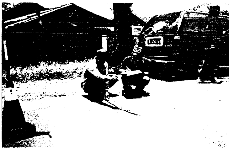
Gambar 2 : Pengukuran lubang ( patching potholes ) dilapangan.
