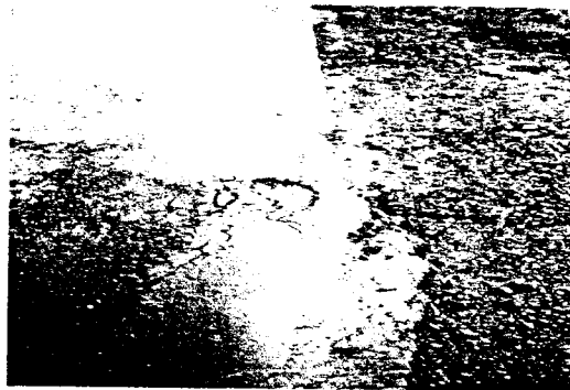
Gambar 2.6: Jembul ( upheaval ).
