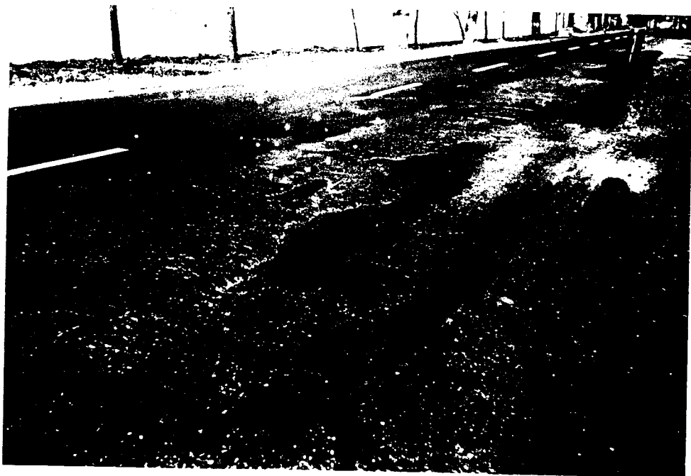
Foto 6. Long&Transversal Cracking
