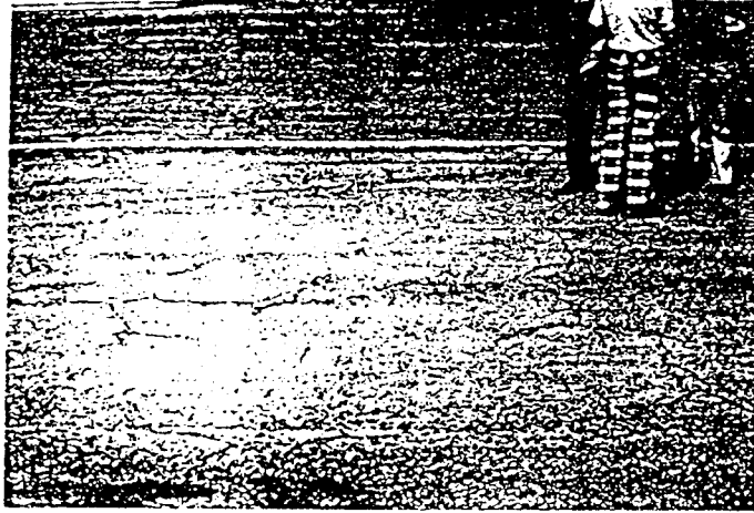
Figure 1-19. Low severity block cracking
