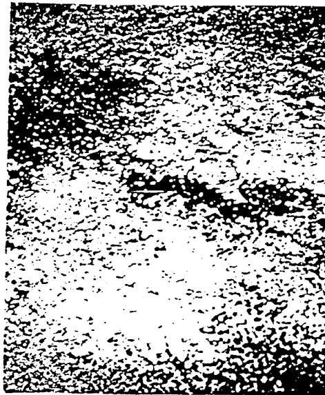
Figure B-54. Medium severity raveling/weathering
