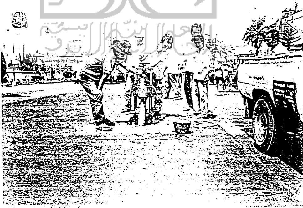
Test Core Drill Aspal Beton
