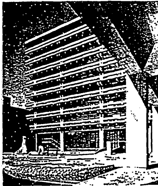
Gambar 2.23 Prefectural Office of Kagawa
