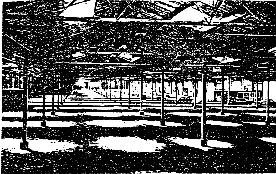
Gambar 2. 13. Ruang-ruang barang pada lantai bawah (Sumber : Design & Construction of Port & Marine Structures, Alanzo DeF. Quinn , Second Edition 1972)
