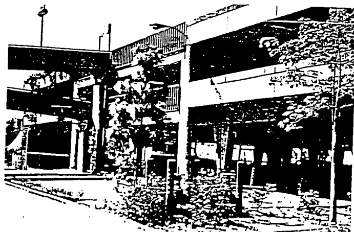
2-31 This parking structure combines precast and poured-in-place concrete construction. Pedestrian skyways lead to the retail portion of the complex.
