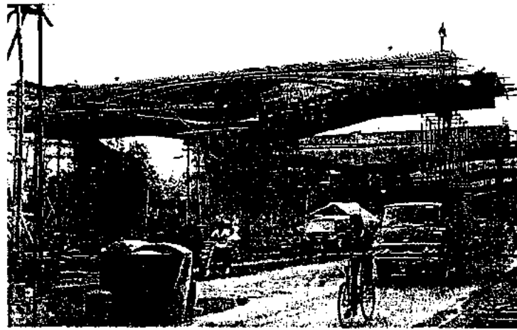
VSL involvement in the 12 km flyover in Cawang - Tanjung Priok toll road (N-S Link). Post-tensioning of piers and beams and launching of beams.
