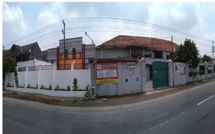
Gambar 4.2 Gedung PT. Globalindo Intimates
