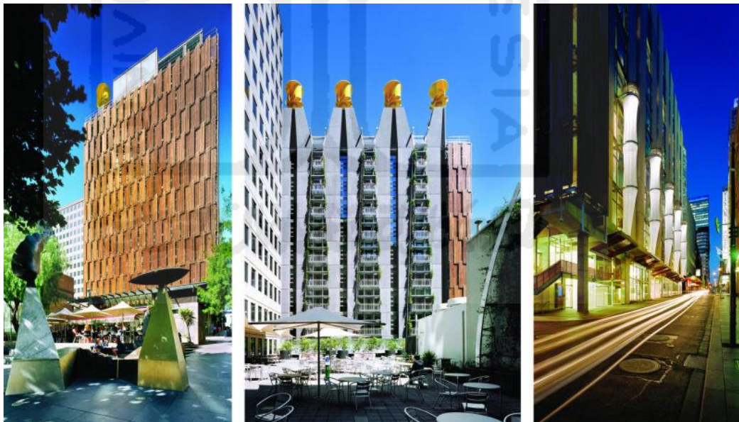
Gambar 34 CH2 Melbourne City Council House 2
