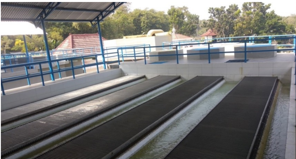
Gambar 4.41 Instalasi SPAM Regional
