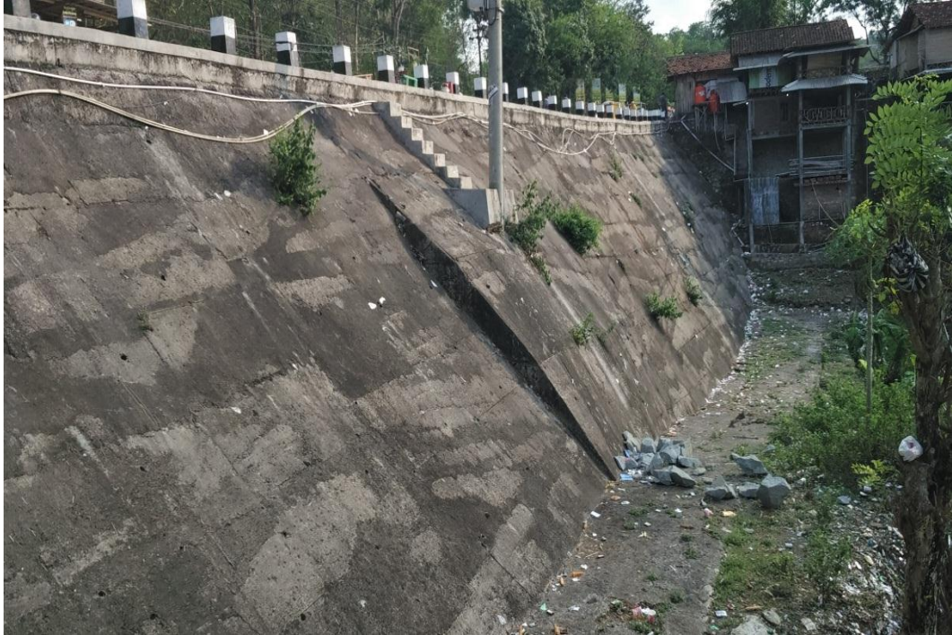
Gambar 5.1 Tampak Dinding Penahan Tanah
