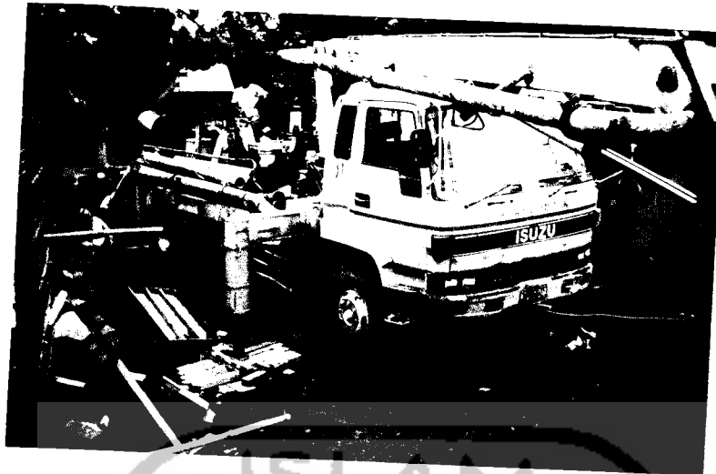
Gambar 4.6 “Ready mix concrete pump truck”
